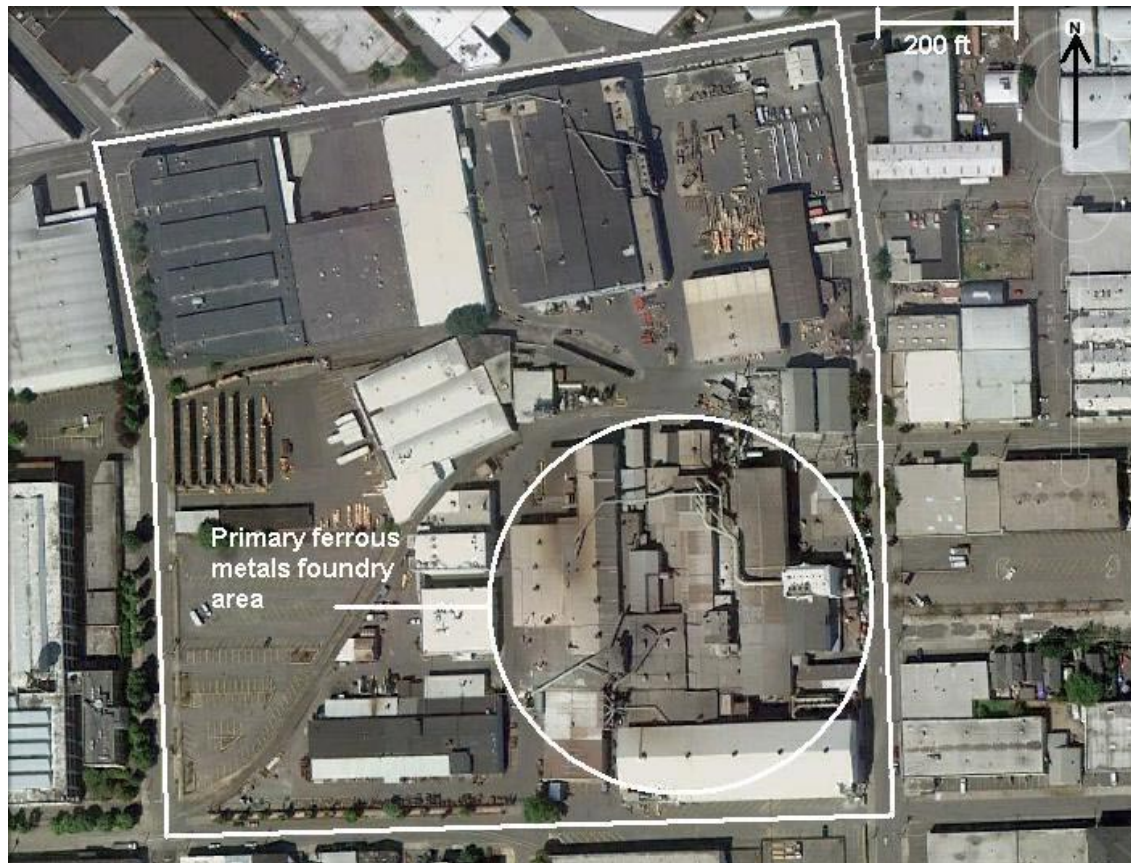
Figure 5. Ferrous Metals Foundry Aerial Map
