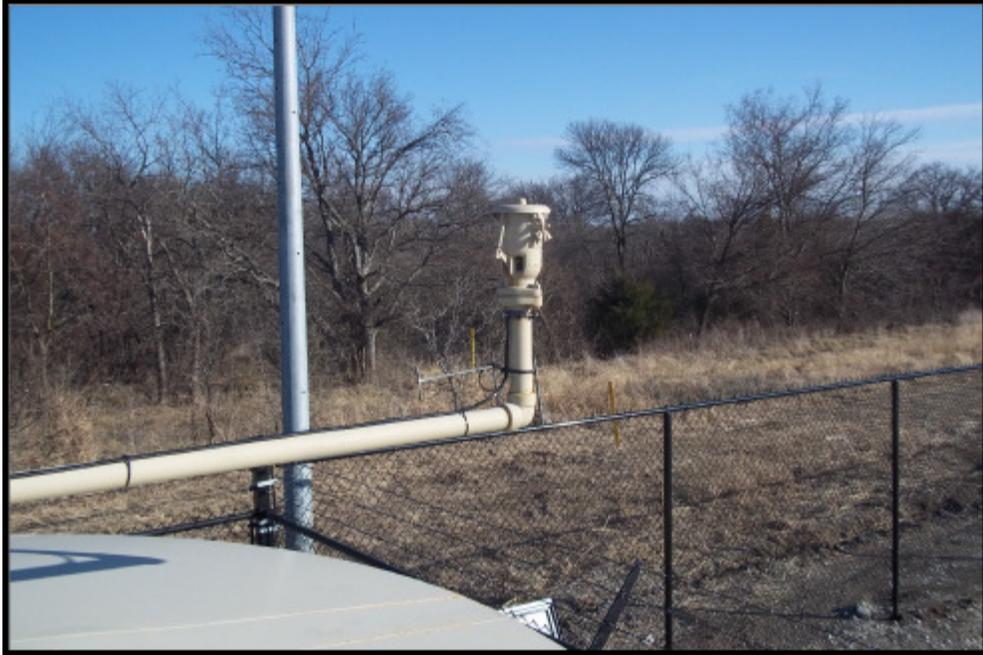
**Figure 4. Storage Tank Vent**
