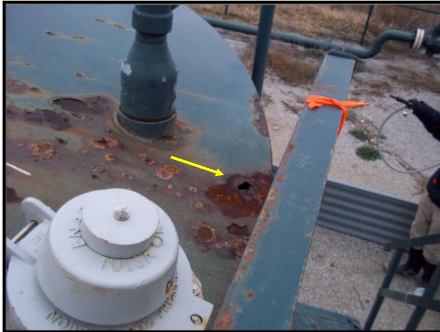
**Figure 6. Hole in Tank Roof - Miscellaneous Emission Source**
