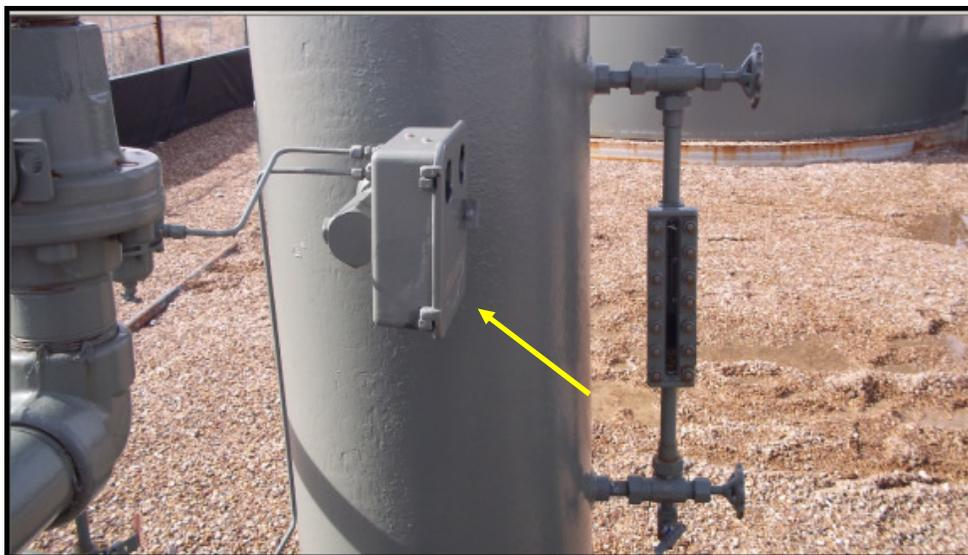
**Figure 3. Pneumatic Valve Controller on Separator**
