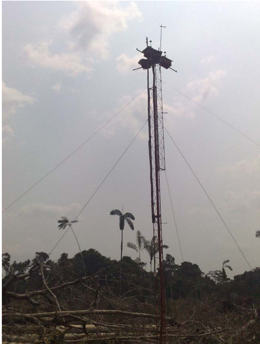
Figure 8 – General view of installed tower.
