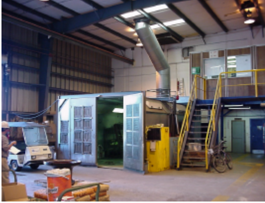
Figure 3. Test Enclosure Prior to Modification
