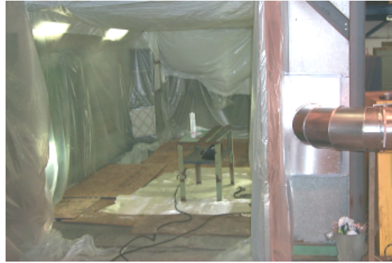
Figure 5. Test Enclosure Interior
