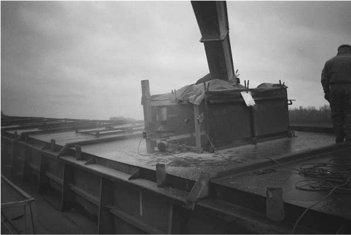
Figure 3. Barge loading test.
