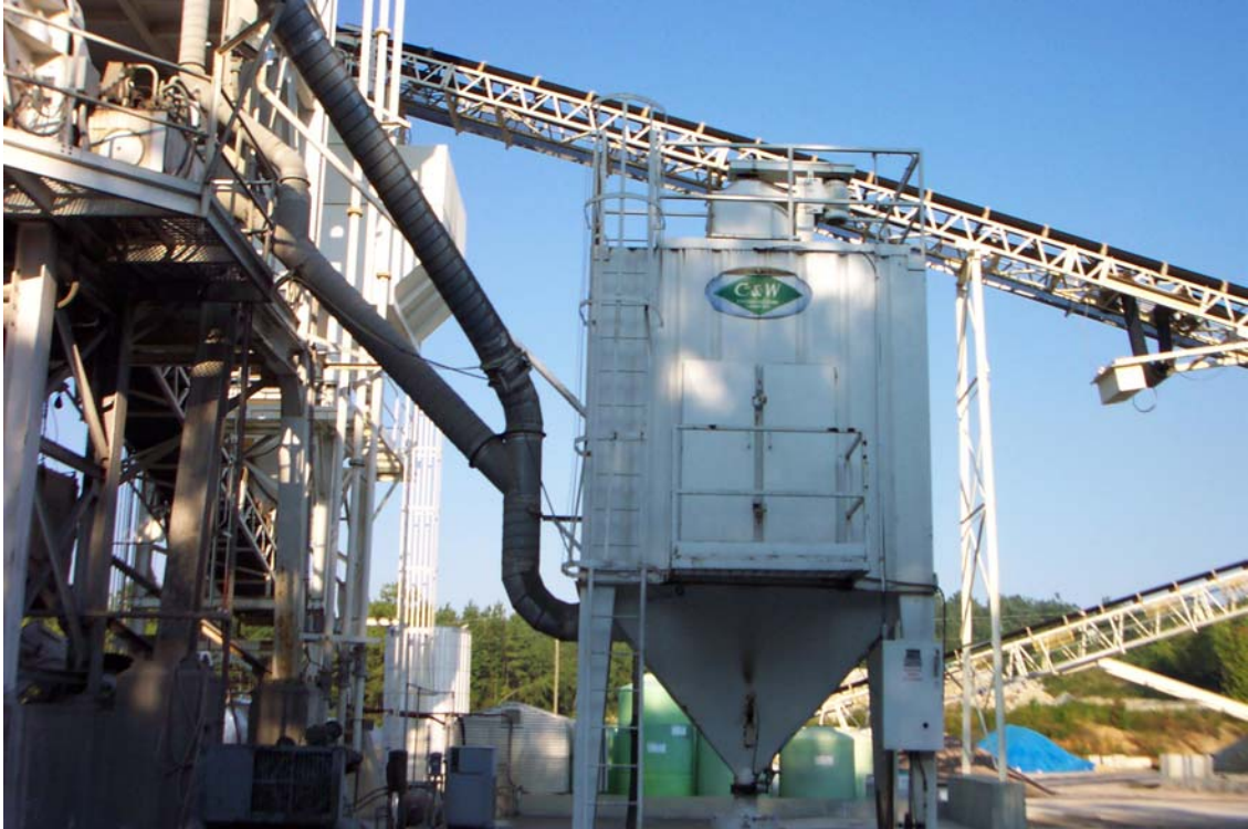
Figure 3-1b. Plant 1 Fabric Filter Inlet Duct Test Location
