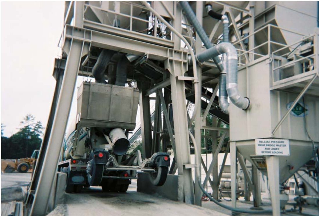
Figure 3-3a. Plant 4 Truck Loading Area
