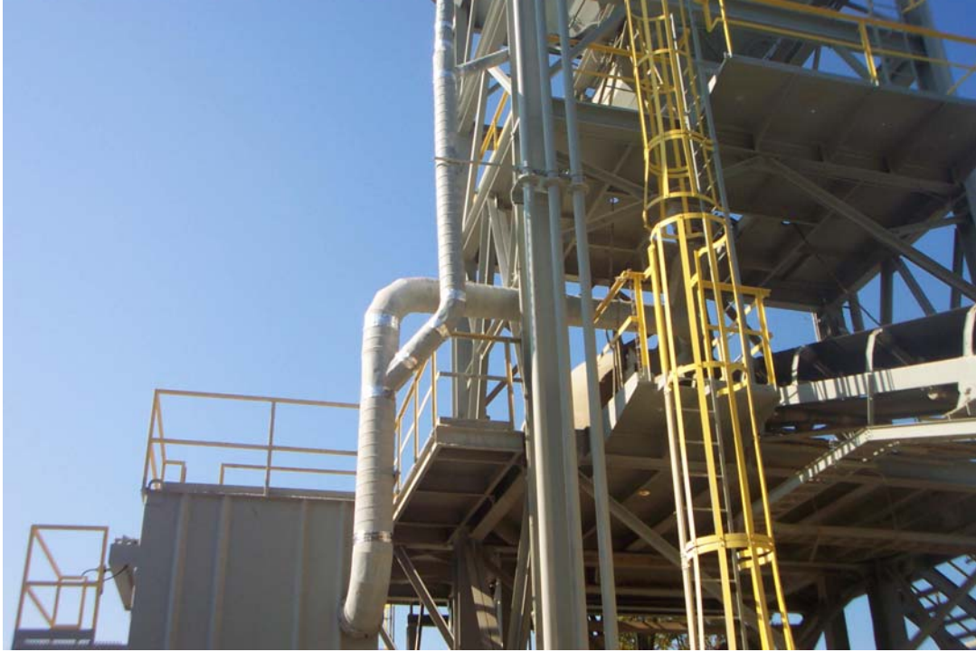
Figure 3-2b. Plant 2 Fabric Filter Inlet Duct Test Location
