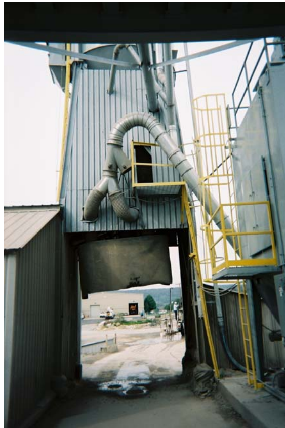
Figure 3.5-a. Plant 6 Truck Loading Area
