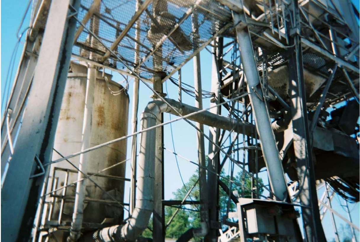
Figure 3-4b. Plant 5 Fabric Filter Inlet Duct Test Location
