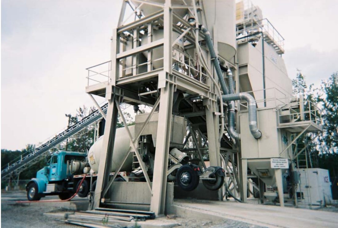
Figure 3-3b. Plant 4 Fabric Filter Inlet Duct Test Location
