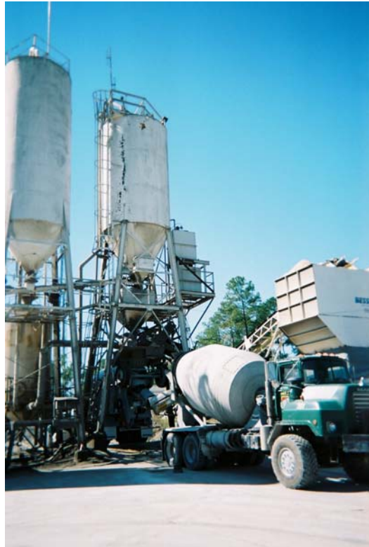
Figure 3-4a. Plant 5 Truck Loading Area
