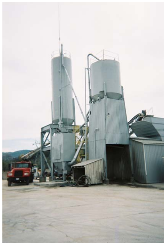
Figure 3-5b. Plant 6 Fabric Filter Inlet Duct Test Location
