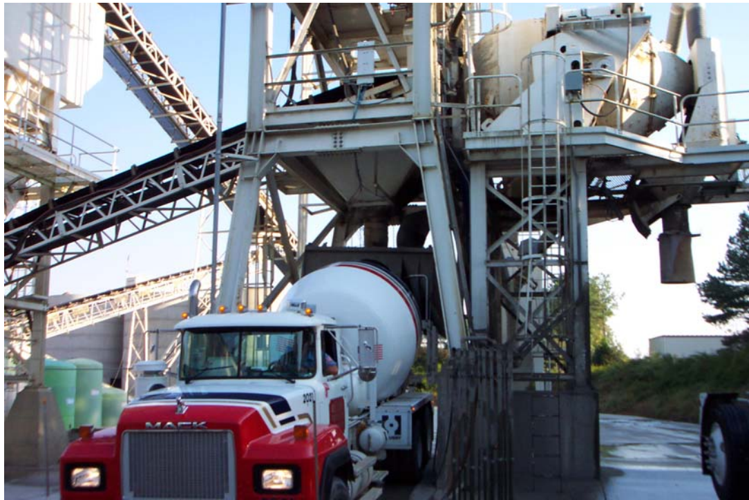
Figure 3-1a. Plant 1 Truck Loading Area
