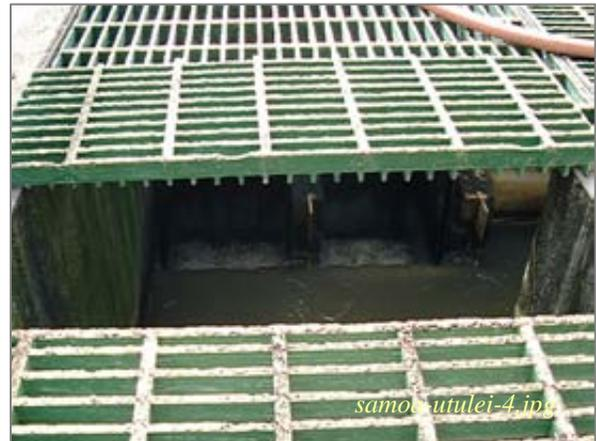
Photo: Utulei STP – Flow Splitter Box
