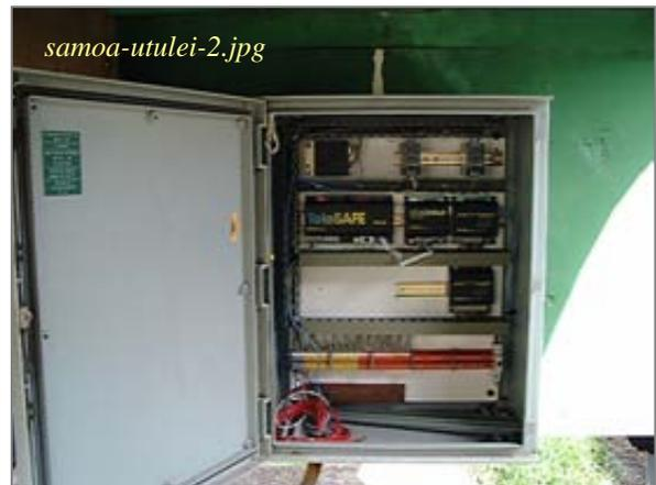
Photo: ASPA Sewers – SCADA Telemetry
