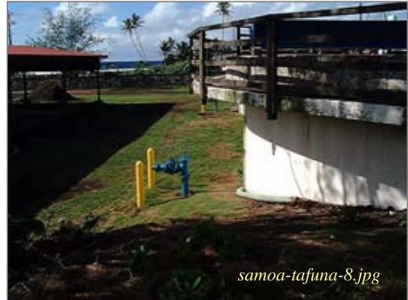
*Photo: Tafuna STP – Sludge Draw-off Valving
