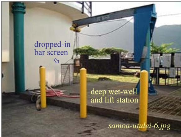
Photo: Utulei STP – Inlet Lift Station
