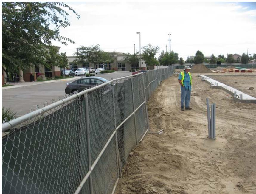
**Photograph 2.** View of the eastern perimeter of the construction site. Note that there is no silt fence to prevent sediment from leaving the site.
