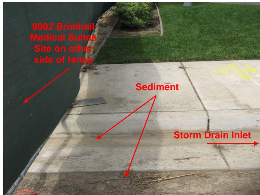
**Photograph 4.** Alternate view of sediment in curb and gutter flow line upgradient of unprotected storm drain inlet shown in Photograph 3. It was not clear to the EPA Inspection Team whether the drain inlet discharged to the City's MS4 or to a retention basin.
