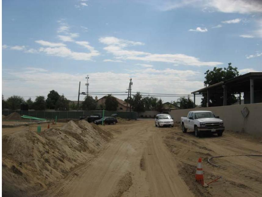
**Photograph 1.** View of southwest corner of the construction site. Note that the site had been initially graded and a contractor was installing building foundation pads at the time of the site visit.
