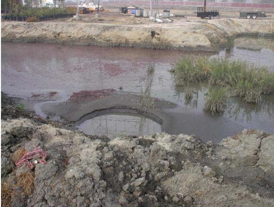
Photo 7: Detention pond in southern corner of yard. Pond is filled with sediment and other debris within about 3-4 feet of the top of the embankment. The pond was apparently recently excavated to remove some of the sediment and debris, which was placed on the embankment (bottom of photo).
