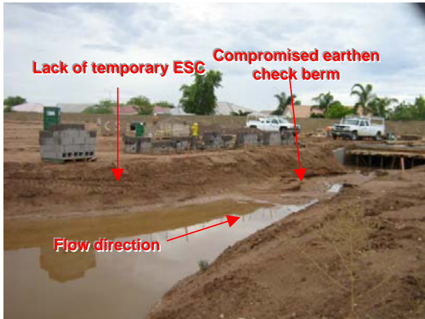
Photograph 4: Mountain View Village Center Lack of temporary ESC between the large expanse of disturbed construction site area and the flowing drainage channel
