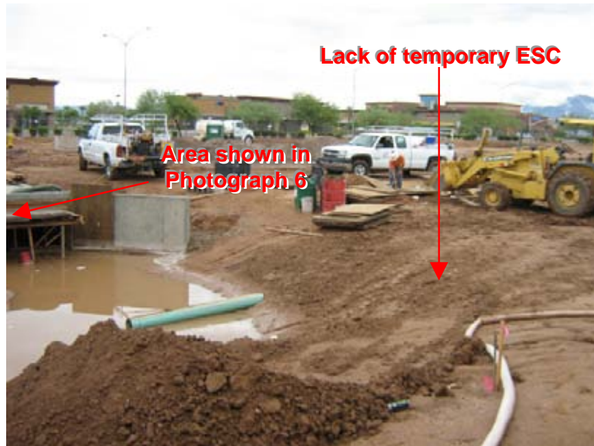
Photograph 5: Mountain View Village Center Lack of temporary ESC between the large expanse of disturbed construction site area and the flowing drainage channel
