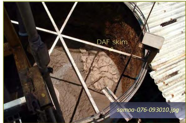
Photo #4: DAF Skim – Holding to High-Strength Tank
