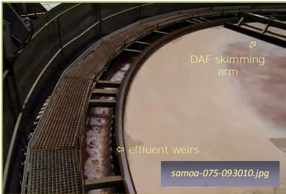
Photo #3: Dissolved Air Flotation Unit – Surface Weirs
