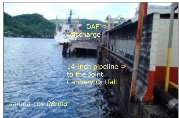
Photo #14: Joint Cannery Outfall Connection Taken By: Greg V. Arthur Date: 04/02/08
