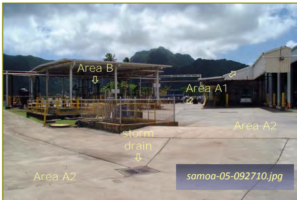
Photo #1-3: Areas A1/A2 - Non-Contact Drainage Taken By: Greg V. Arthur Date: 09/27/10
