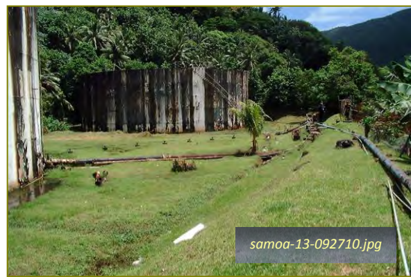
Photo #1-10: Area E - Decommissioned Tanks Taken By: Greg V. Arthur Date: 09/27/10
