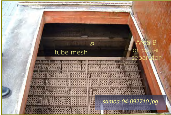
Photo #1-1: Mesh Tube Coalescing Oil Water Sep Taken By: Greg V. Arthur Date: 09/27/10
