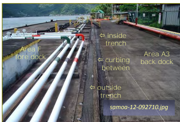
Photo #1-11: Area F/A3 - Fueling Dock Taken By: Greg V. Arthur Date: 09/27/10
