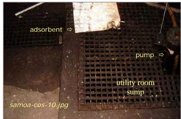
Photo #10: Utility Room Sump - Adsorbent
