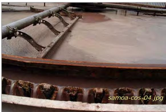
Photo #3: Low-Strength Wastewater - DAF Unit
