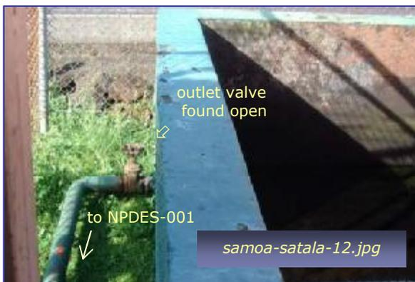
Photo #5: Waste Oil Tanks 2° Containment
