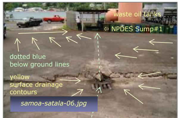
Photo #12: Drainages into NPDES Sump #1
