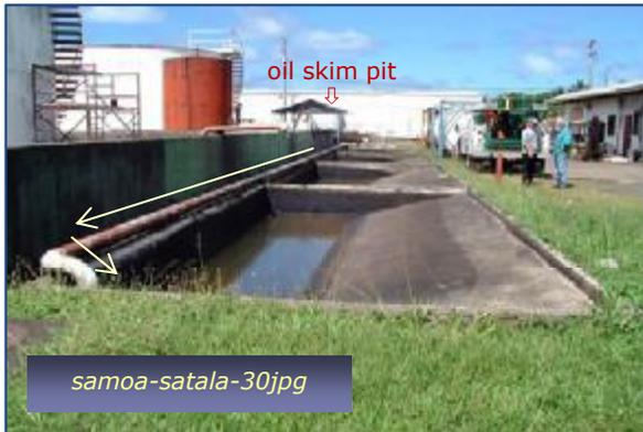
Photo #15: Waste Oil Step 3 - Settling Basins
