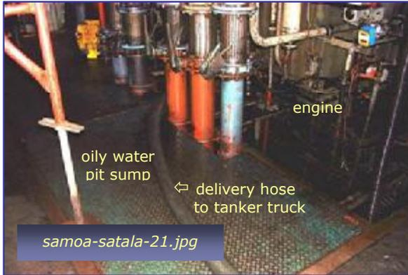
Photo #1: One of Four Power Plant Pit Sumps
