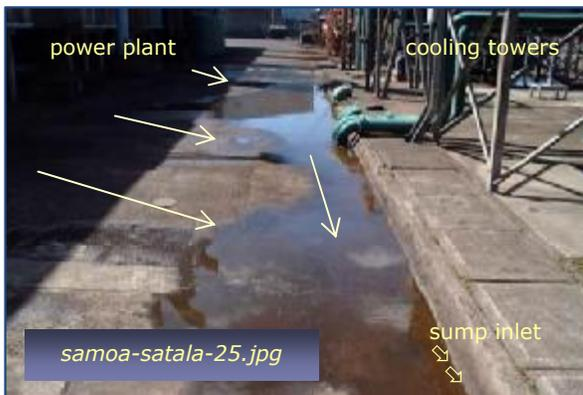
Photo #11: Drainages into NPDES Sump #2
