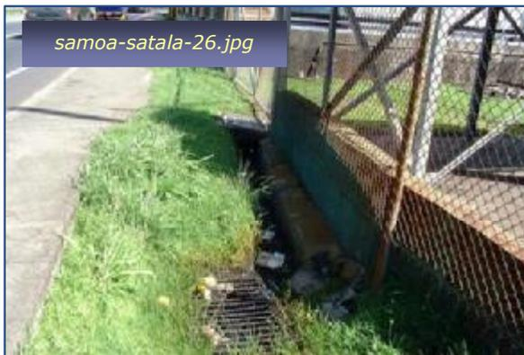
Photo #9: Storm Drainage Ditch – Culvert Inlet
