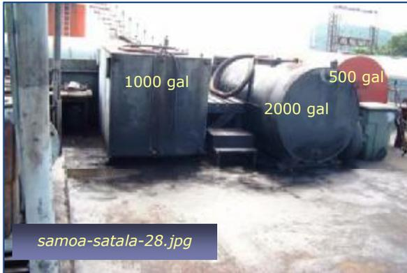
Photo #13: Waste Oil Step 1 - Batch Settling Tanks
