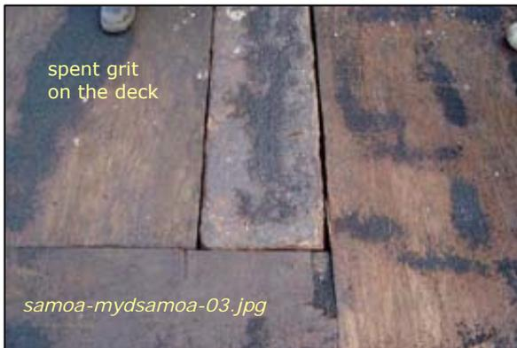
Photo #3: 3000-Ton Dry Dock - Gaps Between Boards
