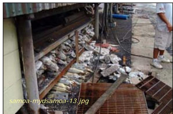
Photo #6: Catch Basin #3 - Zinc Anodes Exposed
