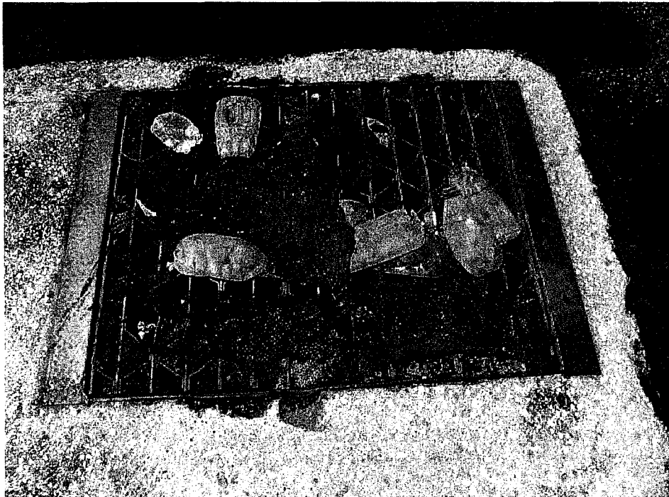
Photo 2 - Close-up of storm drain inlet outside of Horizon Lines maintenance area
