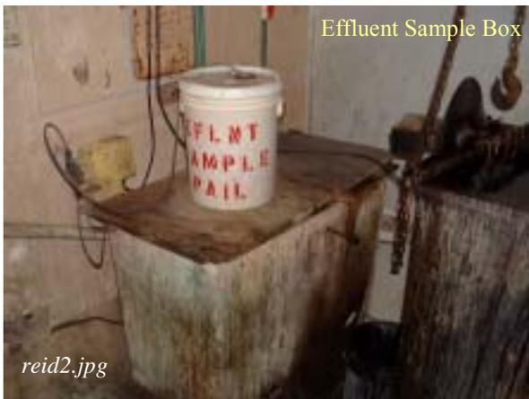
Left shows the effluent sample box (*reid2.jpg*). Reid Metal Finishing collects 24-hour composite samples everyday for internal testing of metals through atomic adsorption.
