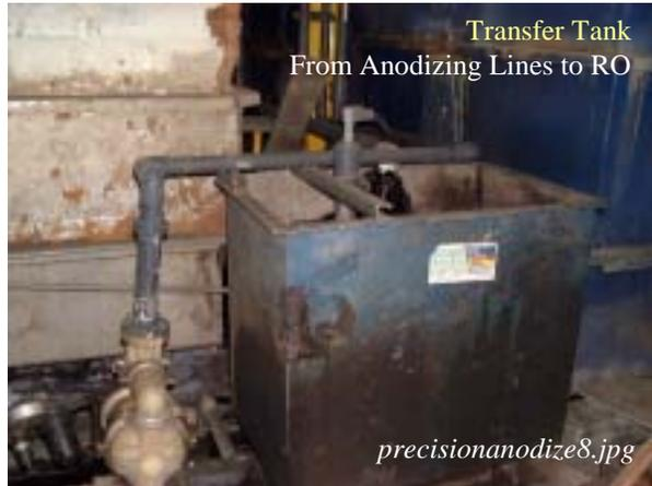
Top left shows the sump pump and spare hoses believed to be used to deliver spents to batch treatment (*precisionanodize13.jpg*). The other three show the three transfer tanks installed to allow the diversion of rinses from the anodizing lines and the zinc-plating line to the RO units for in-plant reuse (~8.jpg, ~9.jpg, and ~11.jpg).
