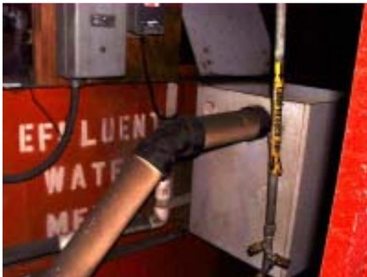
Photo No.4 – Final Metering Tank
