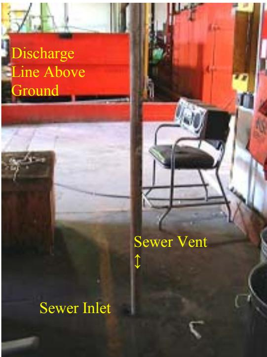
Photo No.2 – Sewer Vent Inlet
