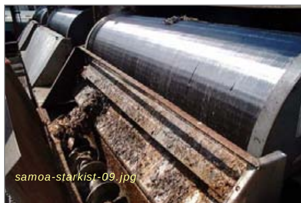
Photo #8: Low-Strength Treatment - Rotoscreens Taken By: Greg V. Arthur Date: 04/03/08
