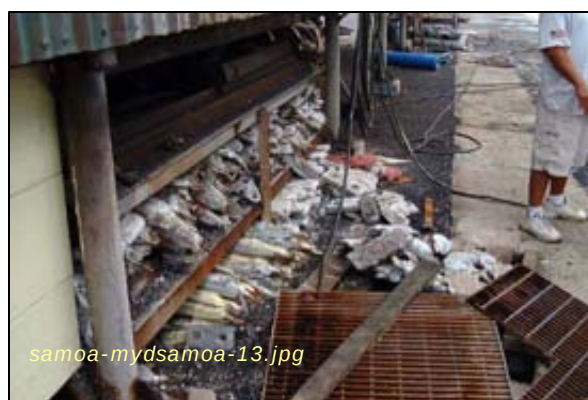
Photo #6: Catch Basin #3 - Zinc Anodes Exposed Taken By: Greg V. Arthur Date: 04/01/08
