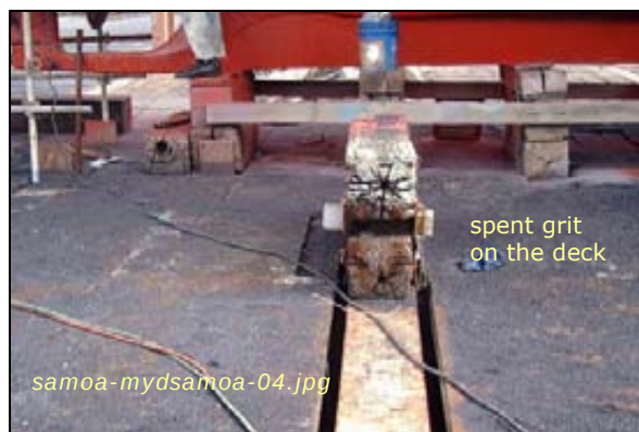
Photo #2: 3000-Ton Dry Dock - Gaps in Decking Taken By: Greg V. Arthur Date: 04/01/08
