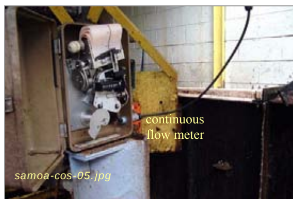
Photo #8: NPDES Sample Point - Flow Meter Taken By: Greg V. Arthur Date: 04/02/08
