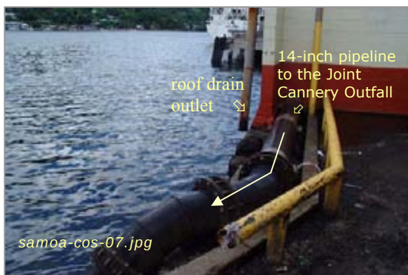
Photo #5: Line to the Joint Cannery Outfall Taken By: Greg V. Arthur Date: 04/02/08
