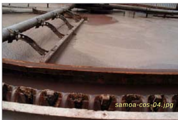
Photo #3: Low-Strength Wastewater - DAF Unit Taken By: Greg V. Arthur Date: 04/02/08
