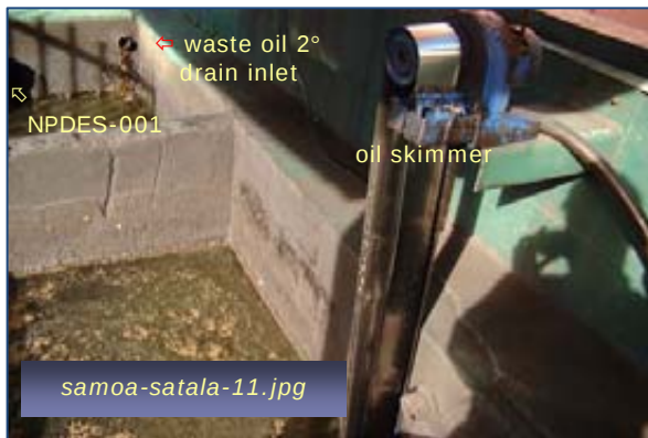
Photo #7: NPDES Sump #1 – Eastern Oil Water Sep Taken By: Greg V. Arthur Date: 04/30/09
