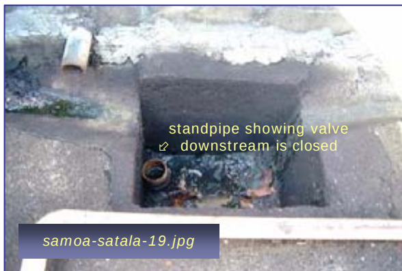
Photo #3: Drainage Sump within Fuel Tank Farm Taken By: Greg V. Arthur Date: 04/30/09
