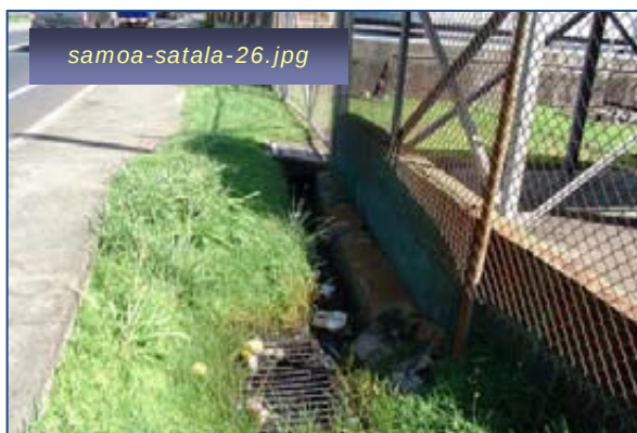
Photo #9: Storm Drainage Ditch – Culvert Inlet Taken By: Greg V. Arthur Date: 04/30/09
