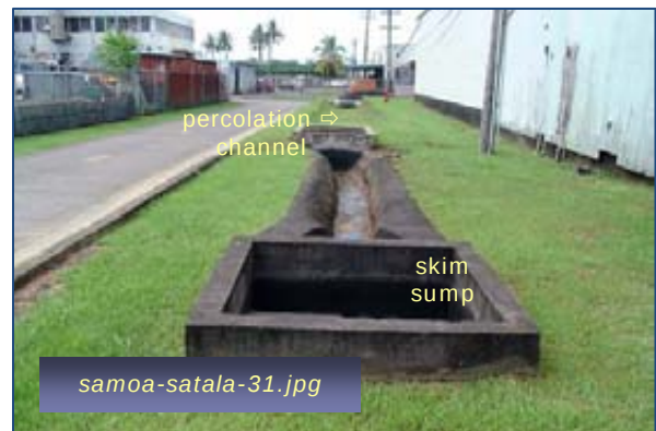
Photo #16: Waste Oil Step 4 - Percolation Taken By: Greg V. Arthur Date: 04/30/09
