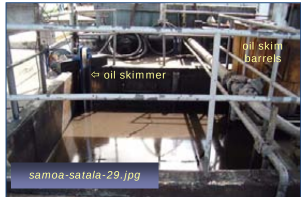
Photo #14: Waste Oil Step 2 - Oil Skim Pit Taken By: Greg V. Arthur Date: 04/30/09
