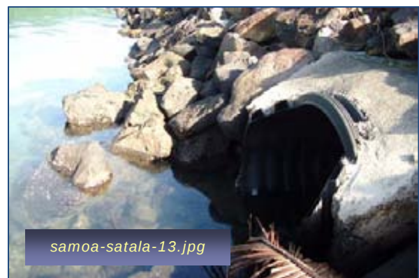
Photo #10: Culvert Outlet to the Harbor Taken By: Greg V. Arthur Date: 04/30/09
