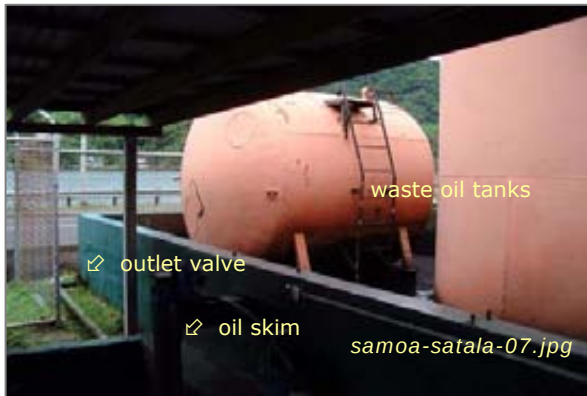
Photo #3: NPDES Sump #1 – Waste Oil Tanks Taken By: Greg V. Arthur Date: 04/01/08
