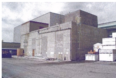
TRA-644, ETR Heat Exchanger Building
