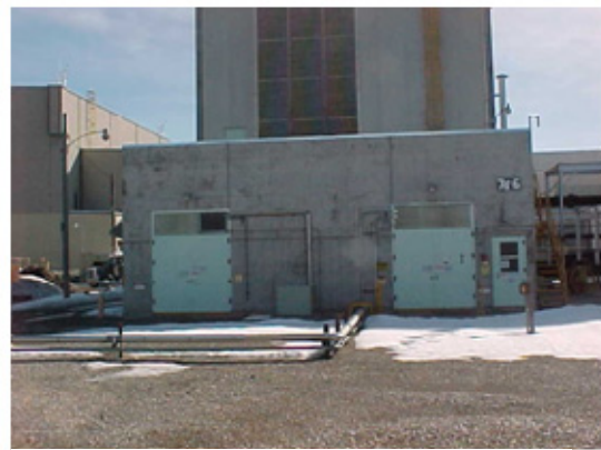
MFC-766, Sodium Boiler Building
