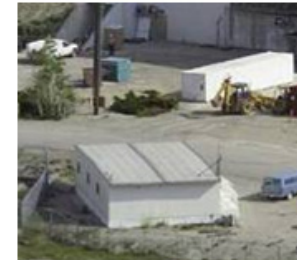
TAN-TR-25, LOFT ICP Support Facility I
