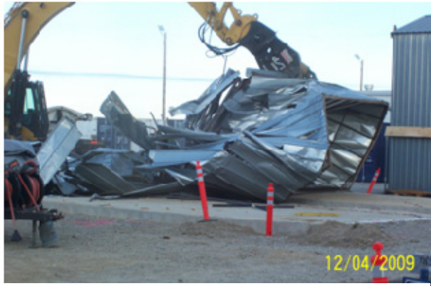
MFC-793E and MFC-793F, Sodium Storage Buildings, with NTCRA underway
