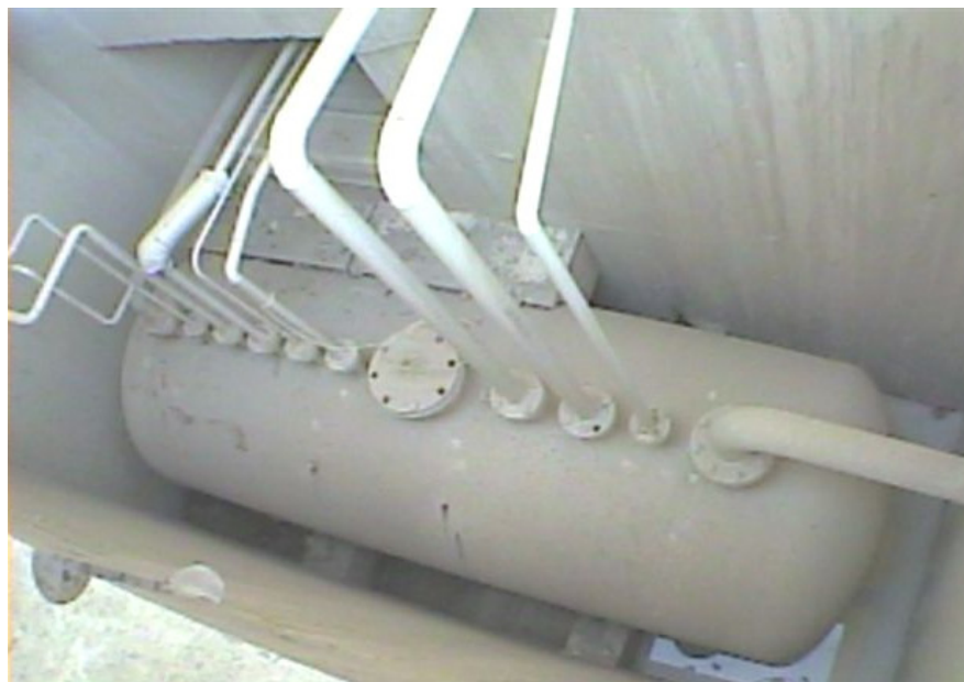
Figure 4-19. SFE-20 tank in vault before removal.
