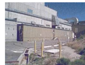
TAN-686, Office Trailer
