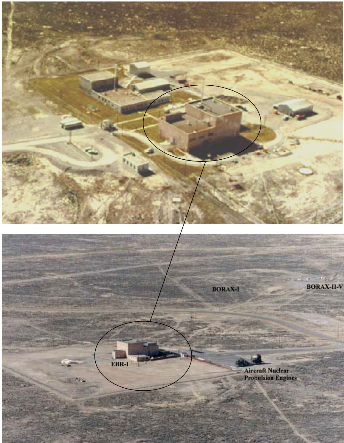
Figure 7-1. Aerial photographs of Experimental Breeder Reactor I before and after decommissioning and the Boiling-Water Reactor Experiment area after decommissioning.
