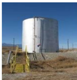
TAN-704, Boiler Fuel Tank
