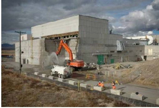
TAN-607A at start of demolition
