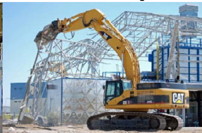
WMF-671, Glovebox Excavator Method Weather Enclosure Structure, before, during, and after decommissioning
