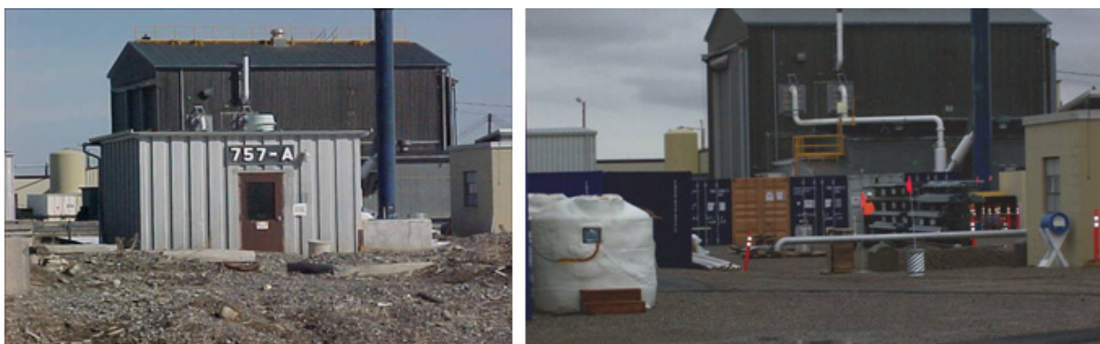
MFC-757A, Cooling Tower System Building, before and after NTCRA
