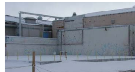
CPP-627, Remote Analytical Facility, slab after demolition
