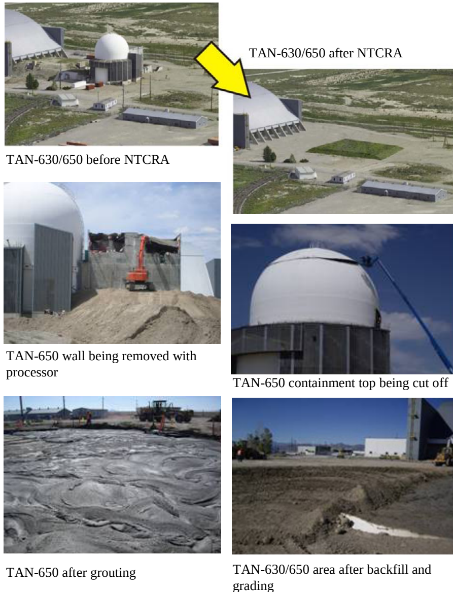
Figure 2-18. Photographs of TAN-630/650 non-time-critical removal actions.
