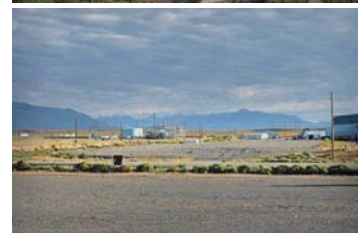
WMF-714 Intermediate-Level Transuranic Storage Facility Pad #1 before, during, and after decommissioning
