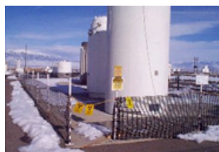
TAN-791, Spent Fuel Storage Pad
