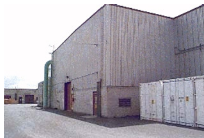
TRA-643, ETR Compressor Building
