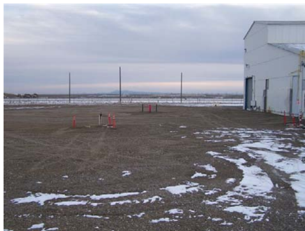
Figure 4-21. Finished grade at the SFE-20 site.
