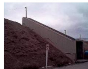
TAN-727, Covered Stairs
