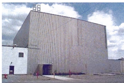
TRA-642, Engineering Test Reactor Building
