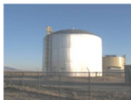
TAN-733, Water Storage Tank
