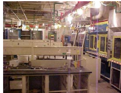
CPP-627, Remote Analytical Facility, shift laboratory
