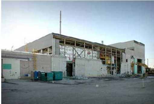
TAN-607A walls being removed
