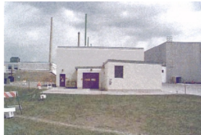
TRA-632, Hot Cell Building
