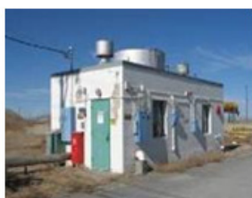
TAN-611, Fuel Pump House
