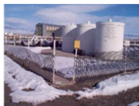
TAN-790, Abnormal Waste Storage Pad
