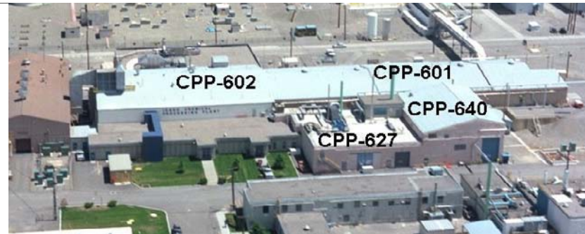
CPP-627, Remote Analytical Facility pre-decommissioning
