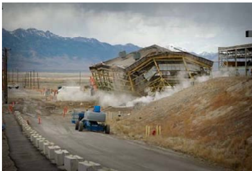
TAN-607A structure coming down
