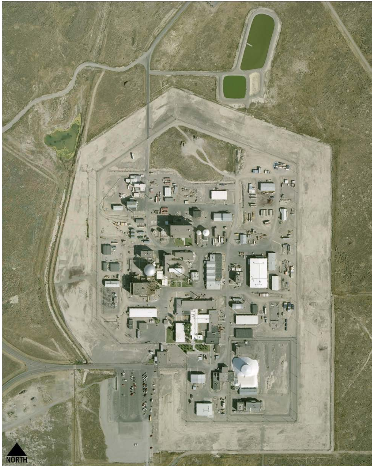
Figure 9-1. Aerial photograph of the Materials and Fuels Complex.
