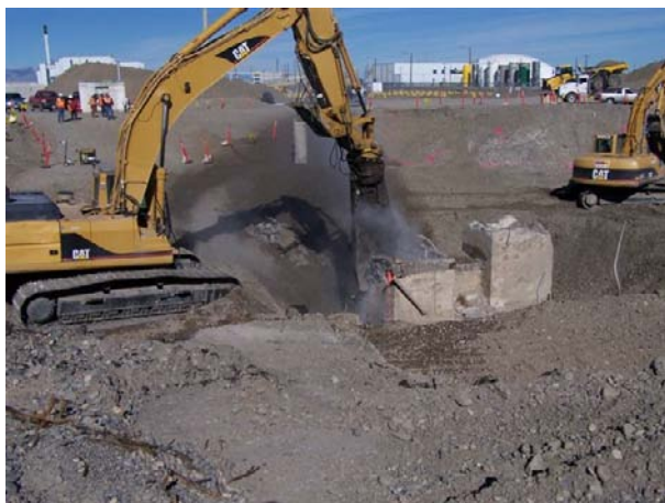
Figure 4-20. Demolition of the SFE-20 vault.
