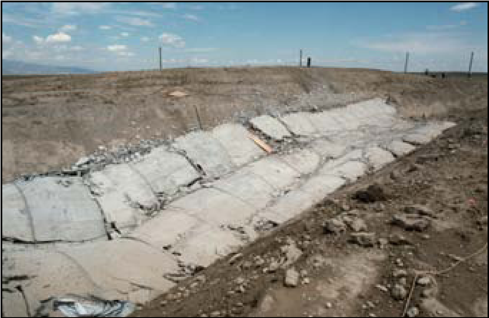
Figure A-5. Photo of the horizontally collapsed Initial Engine Test stack in trench (IAEA 2005).
