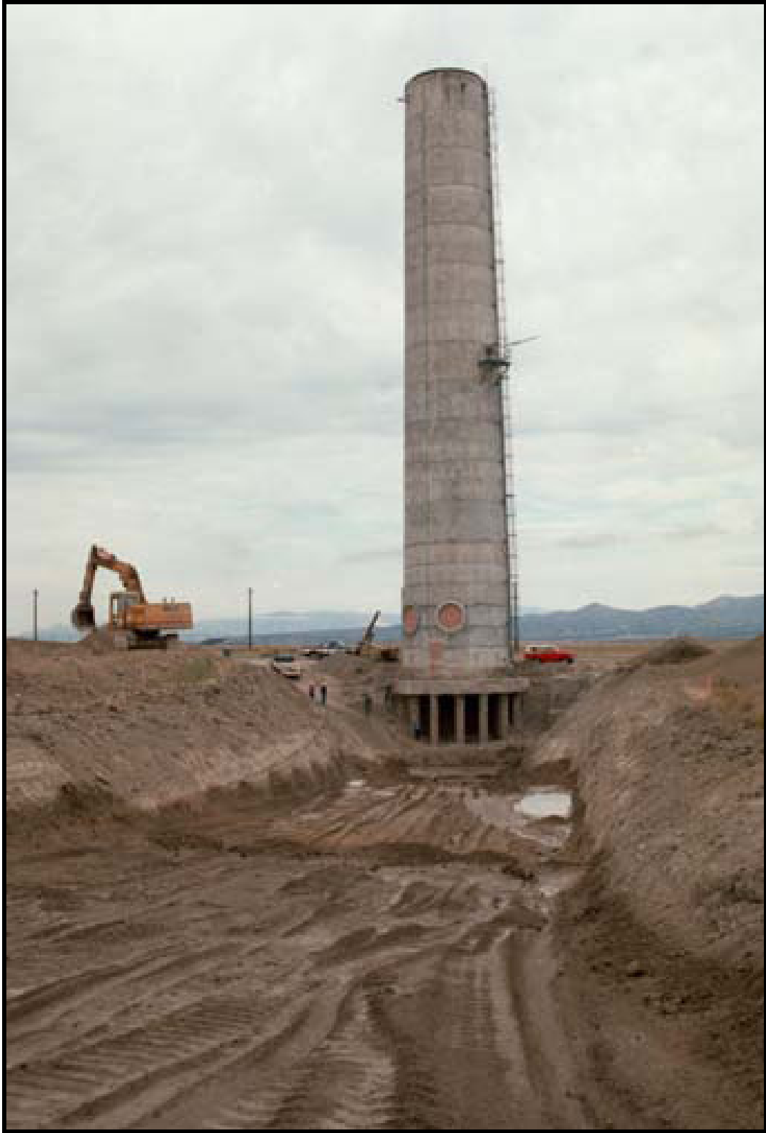
Figure A-4. Photo of the Initial Engine Test stack showing excavated base, supports, and trench (IAEA 2005).
