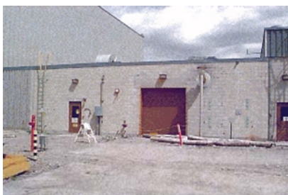
TRA-648, ETR Electrical Building
