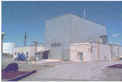
PBF-620, Reactor Building, before NTCRA
