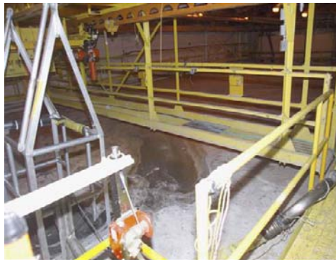
CPP-603A Wet Fuel Storage Facility Basin, south basins after grouting
