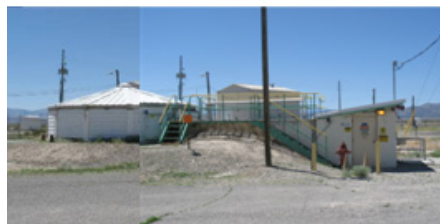
TAN-711, Sewage Treatment Plant; TAN-623, Sewage Pump House
