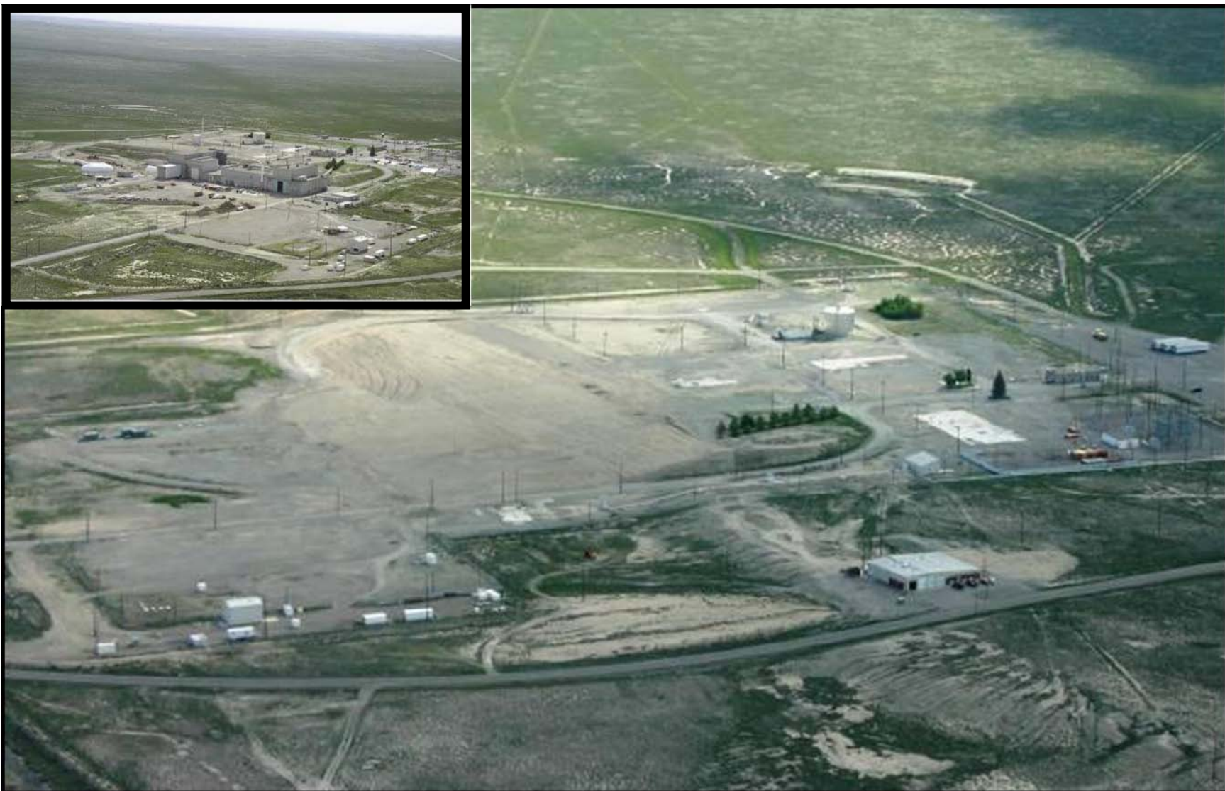
Figure 2-16. Photograph of Test Area North Technical Support Facility before (upper left) and after deactivation and decommissioning activities.
