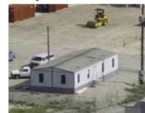
TAN-TR-26, LOFT ICP Support Facility II
