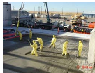
CPP-627, Remote Analytical Facility, slab being reinforced
