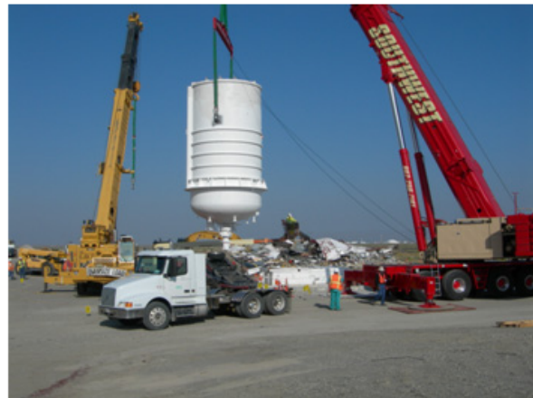
PBF-620 reactor vessel being lifted
