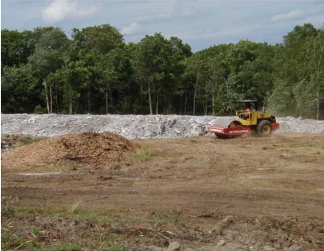
**Waste consolidation at SWA (lime-based Posi-Shell™ is sprayed on piles to reduce odors)**
