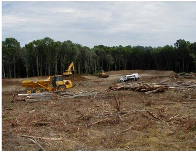
**Site preparation for the future SWA “constructed wetlands” and stormwater retention system**
