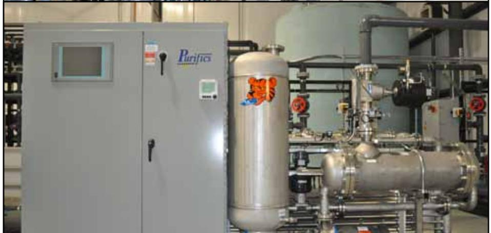
*(Fig.3a - above) Landfill Area treatment system (Fig.3b - below) UV Oxidation unit destroys contamination*
