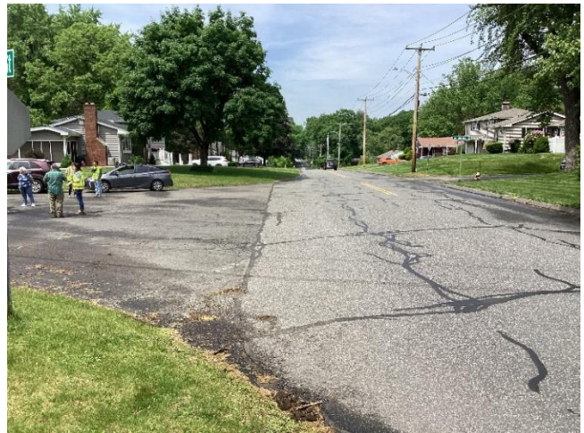
Grandview Street at Hillside Avenue
