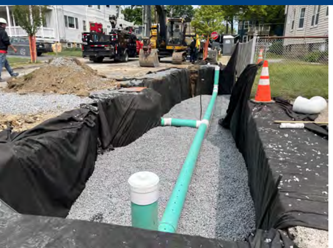
Gravel Reservoir/Underdrain of Tree Trench (Credit: HW)
