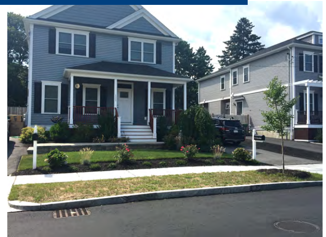
Completed Installation of Tree Trench (Credit: HW)
