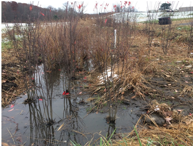
Figure 6. Clogging of bioretention media with silage and sediment.
