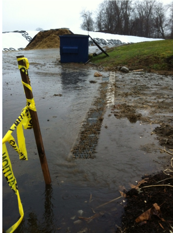
Figure 7. Trench drain clogged with silage debris.
