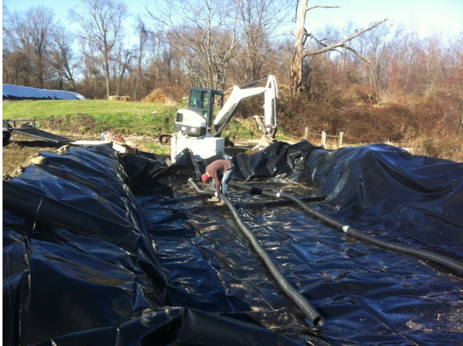
Figure 1. Installation of liner beneath bioretention unit, Storrs, CT.
