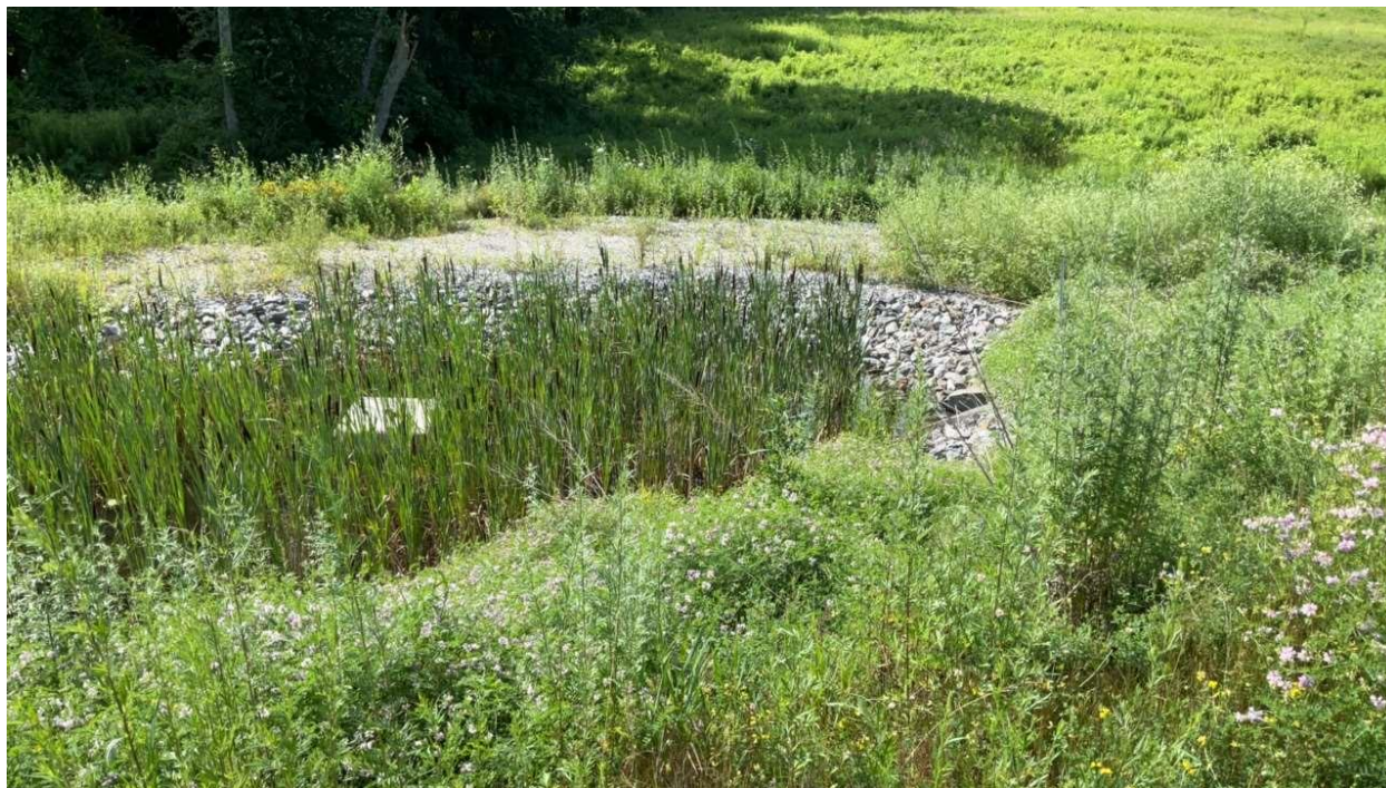
An example of a well-maintained forebay to a treatment facility in Bedford NH, which discharges to BOWMAN BROOK.
