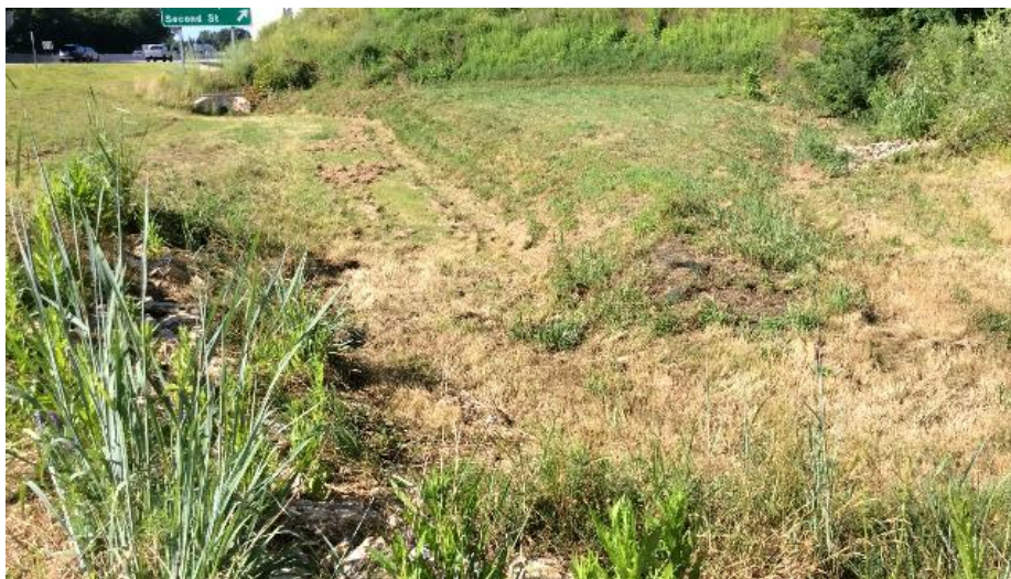
An example of a well maintained vegetated treatment swale in Manchester NH, which discharges to the MERRIMACK RIVER (NHRIV700060803-14-02)
