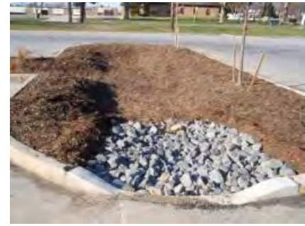
Figure 10. Infiltration Basin (University, 2011)
