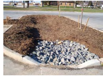
Figure 10. Infiltration Basin (University, 2011)
