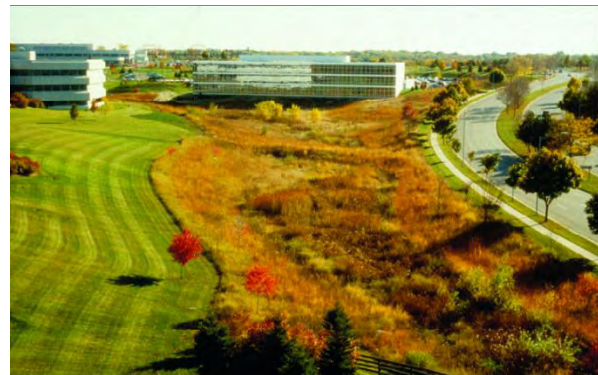
Figure 7. Bioswale (Service, 2005)
