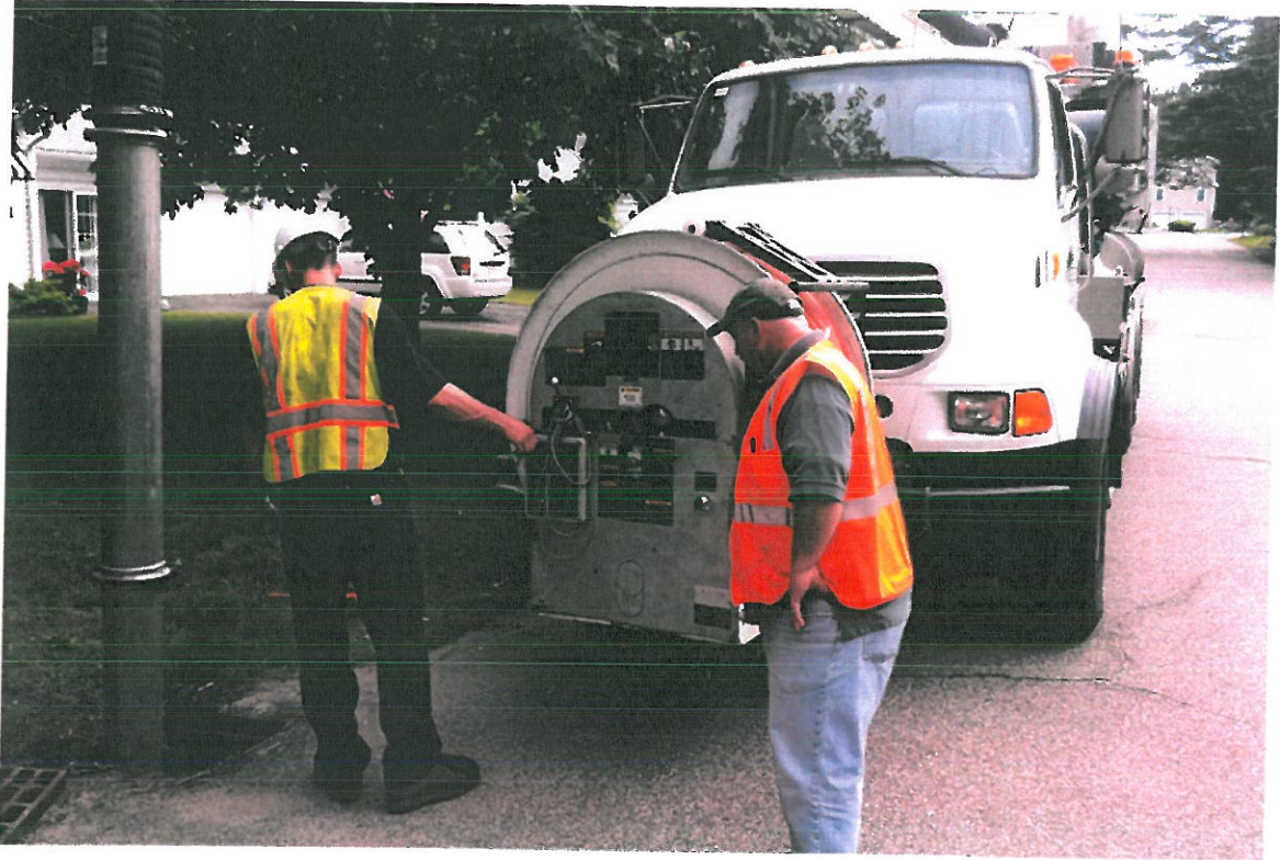
CLEANING CATCH BASINS
