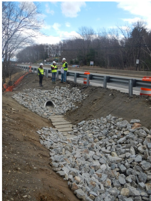
Photo 2. Constructed Infiltration Swale
