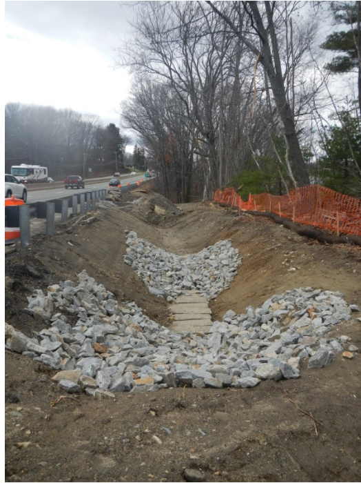
Photo 1. Constructed Infiltration Swale
