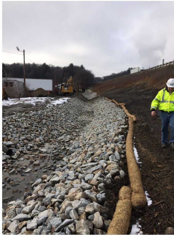
Photo 1. Constructed Infiltration Swale
