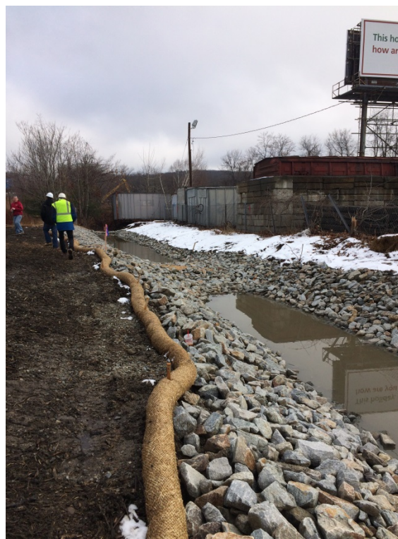
Photo 2. Constructed Infiltration Swale
