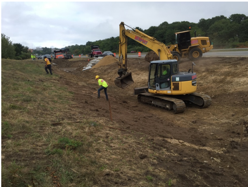
Photo 2. Construction of an Infiltration Swale
