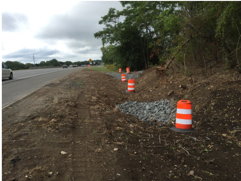
Photo 1. Construction of an Infiltration Swale
