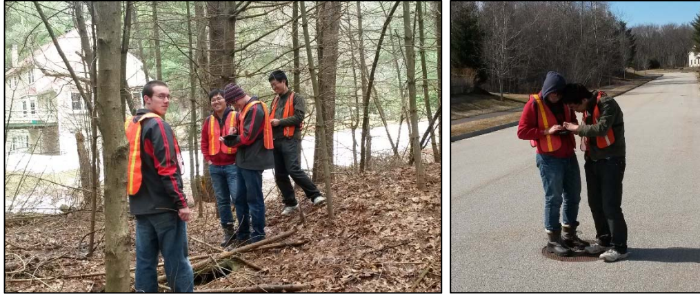
Figure 2: The Coalition's Spring 2014 WPI IQP Student Team Inspecting and Mapping Stormwater Infrastructure in Upton, MA
