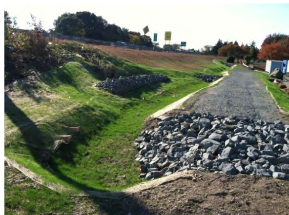
Construction of Infiltration Basin
