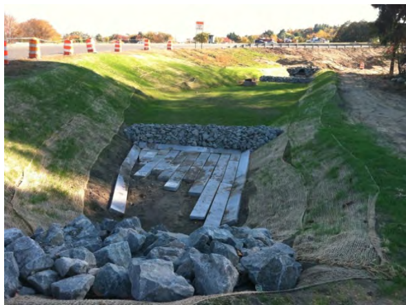
Construction of Infiltration Basin
