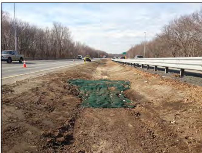
Infiltration swale in I-290 Median
