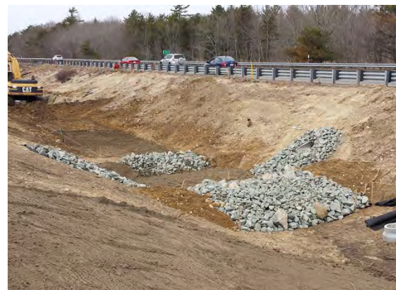
Construction of Infiltration Basin Forebay
