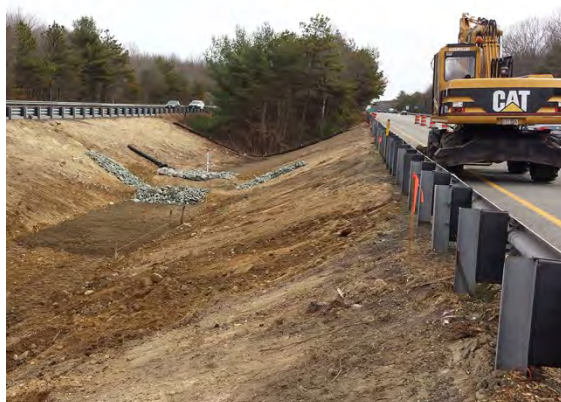
Construction of Infiltration Basin
