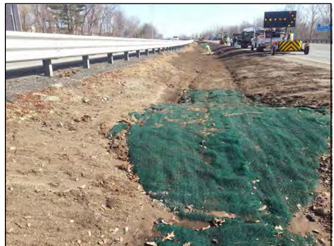
Infiltration swale in I-290 Median
