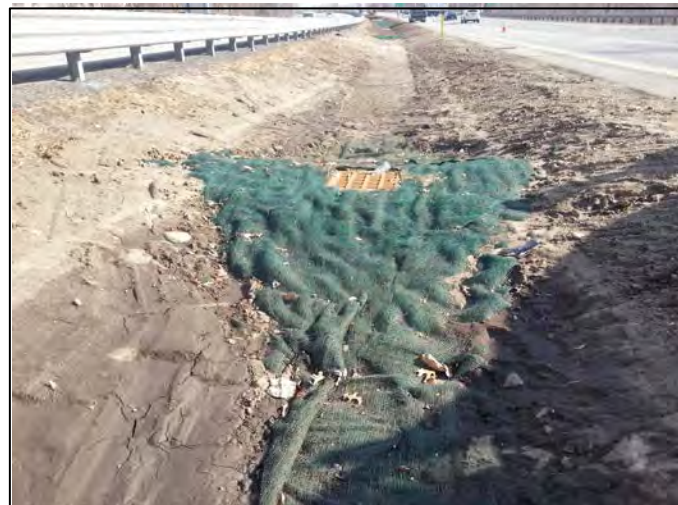
Infiltration swale in I-290 Median
