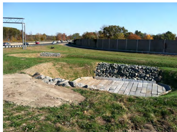
Construction of Infiltration Basin Forebay
