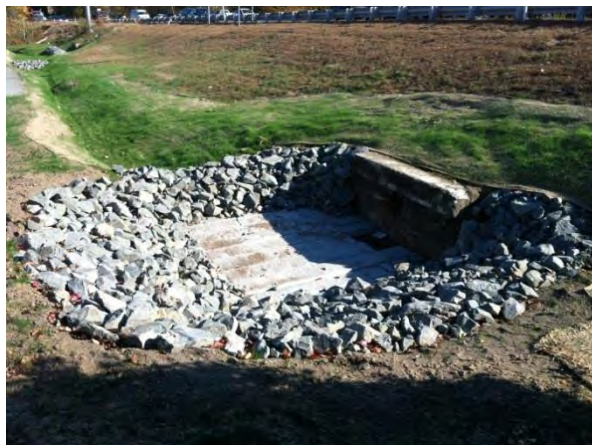
Construction of Infiltration Basin Forebay
