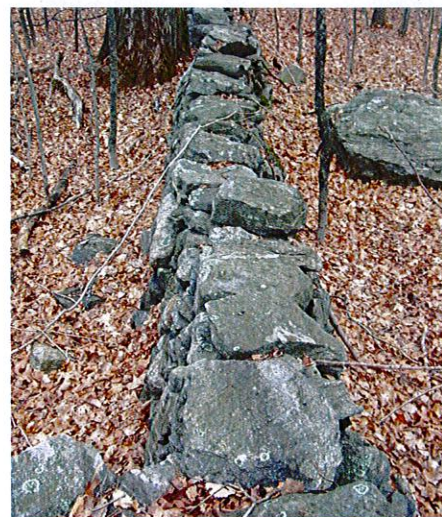
The more carefully constructed "stacked wall" was built to endure the ravages of time, and very likely used to de-mark a property boundary.
