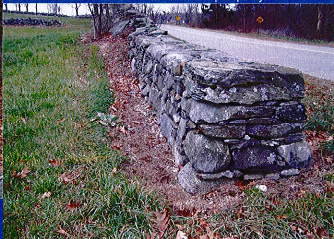
Above is an ideal example of a "filled wall." Two outer walls retain space in between which is filled with stones and debris that erupted from the soil over successive years of use.
