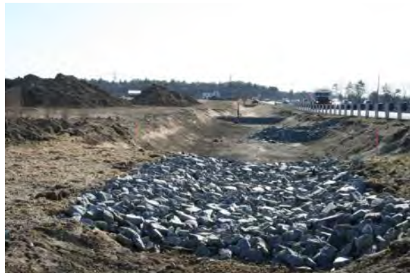
Construction of Infiltration Basin
