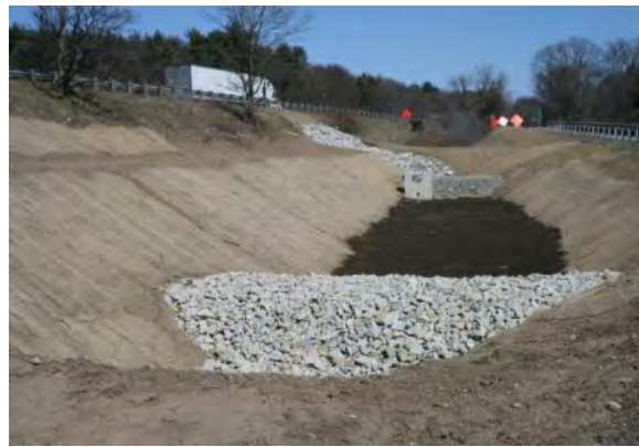
Construction of Infiltration Basin
