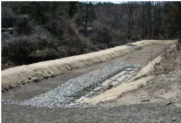
Construction of Infiltration Basin
