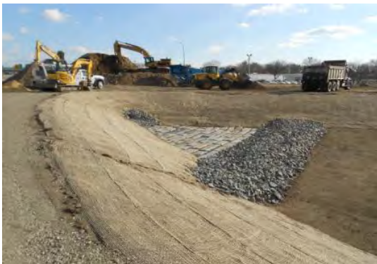
Construction of Infiltration Basin
