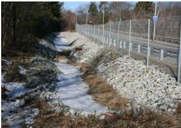
Construction of Infiltration Basin
