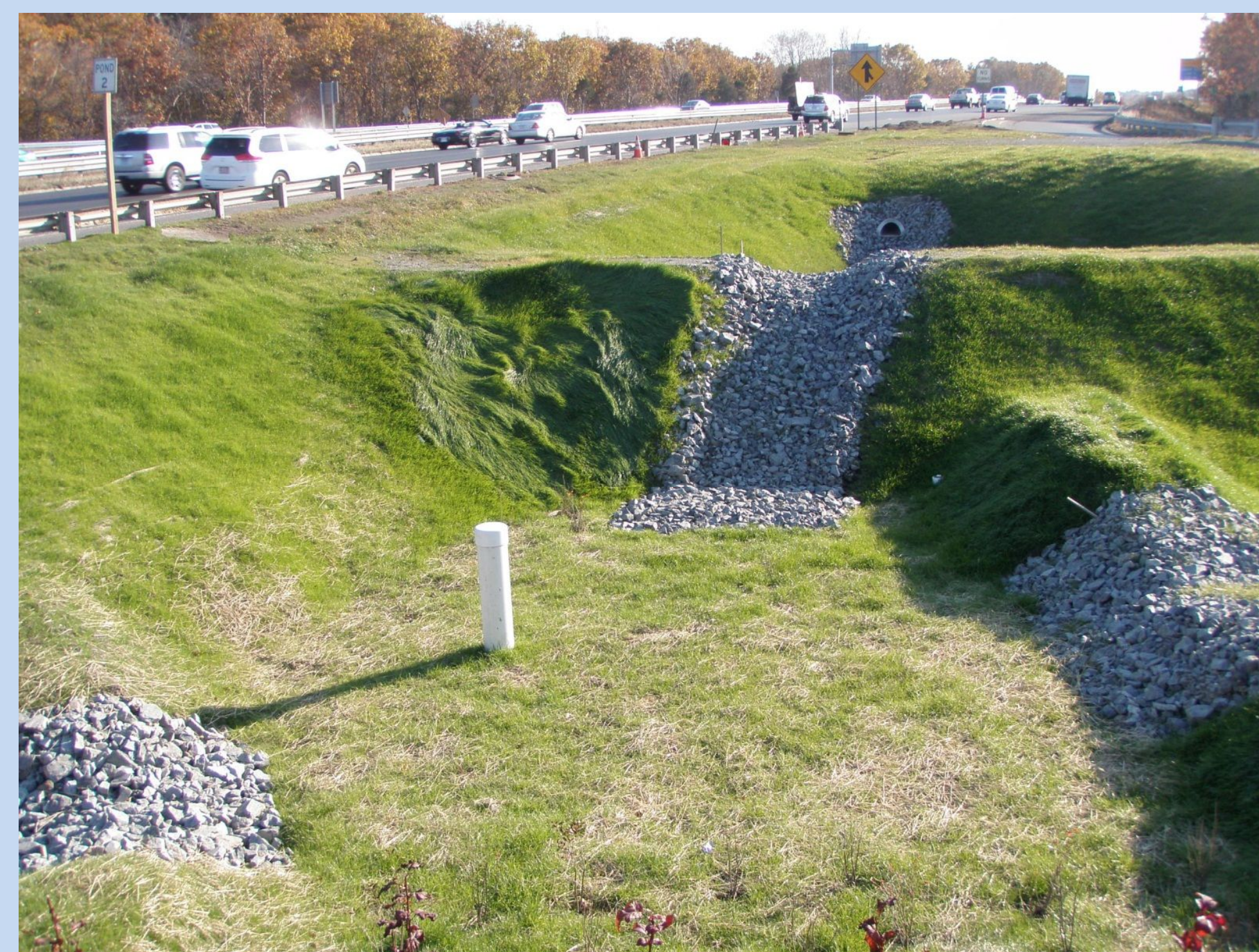
Gravel wetland for stormwater run-off along Rt. 128
