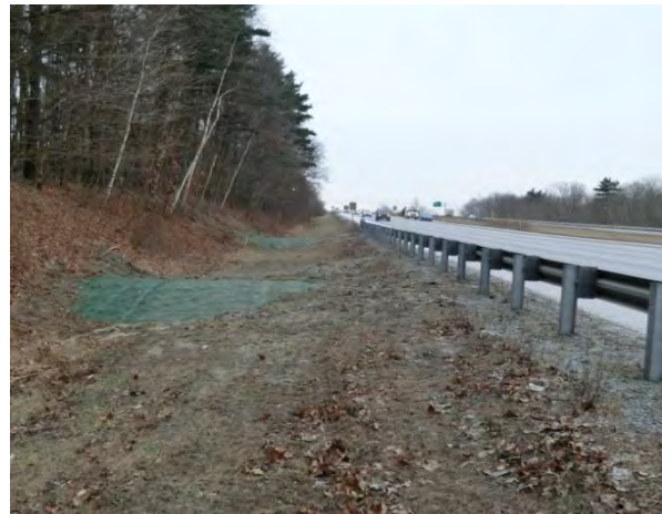
Construction of Infiltration Swale
