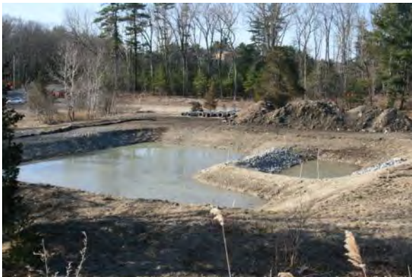
Construction of Infiltration Basin
