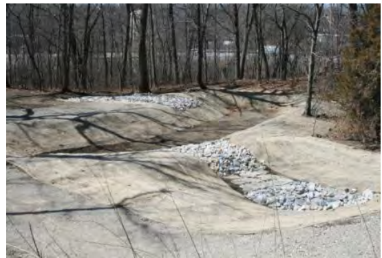
Construction of Infiltration Basin
