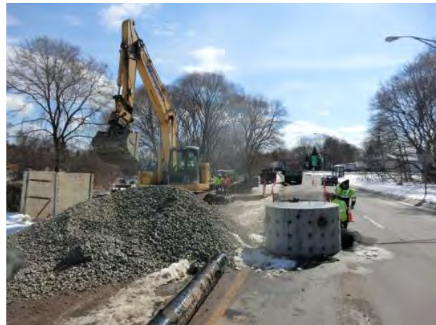
Construction of Leaching Catch Basin
