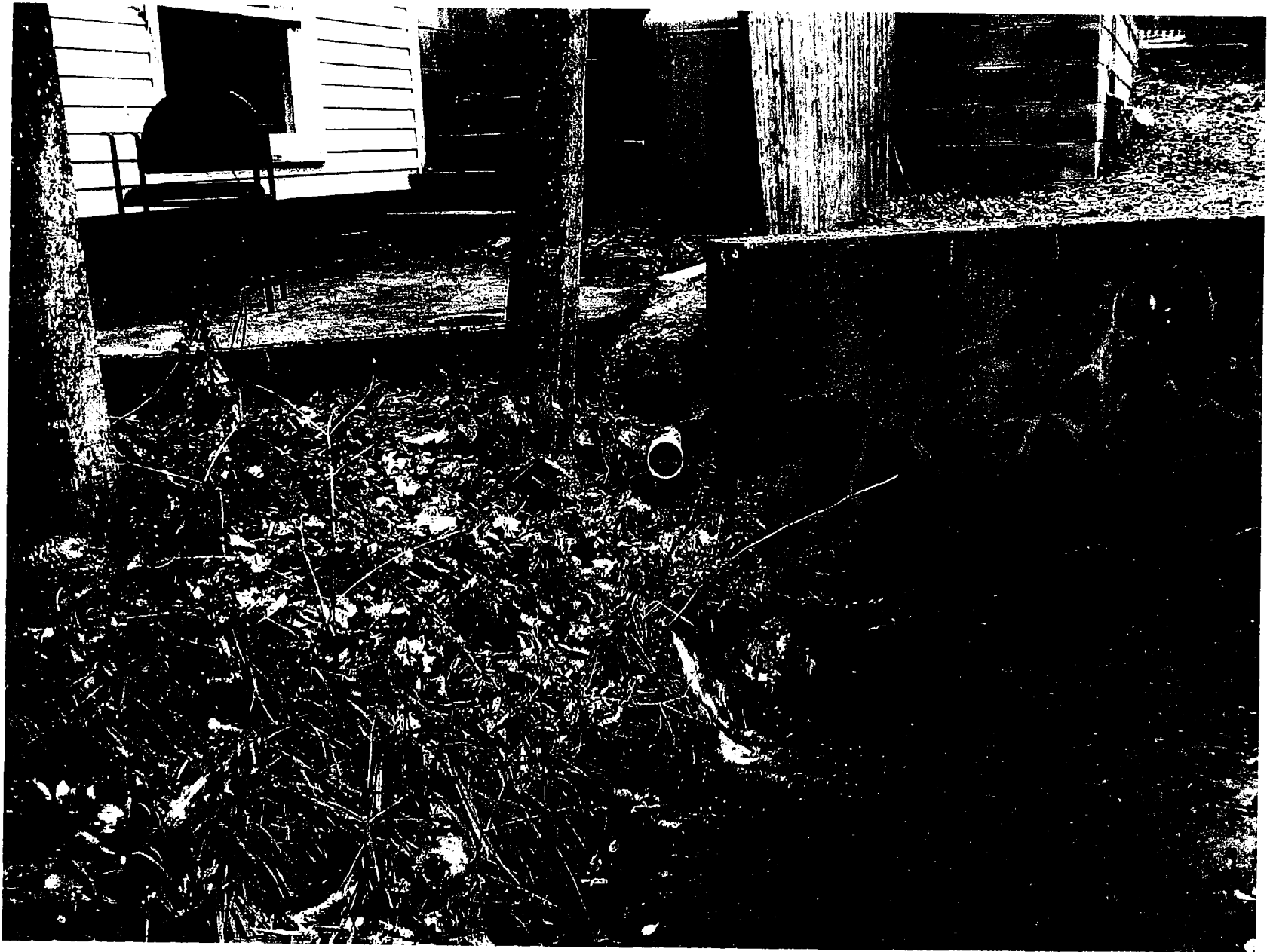
Figure B-14: Outfall #20 and #21
