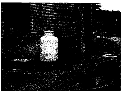
Figure 2-7 Propane tank on east side of Power Plant.
