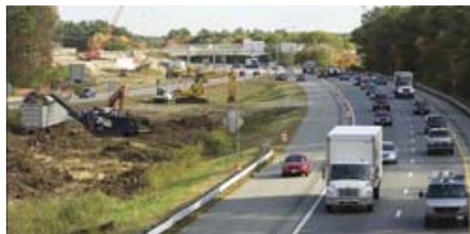
*With University of New Hampshire Stormwater Center support, the New Hampshire Department of Transportation constructed two pilot gravel wetland treatments to help meet TMDL requirements for impaired waters as part of the Interstate 93 widening project.*
