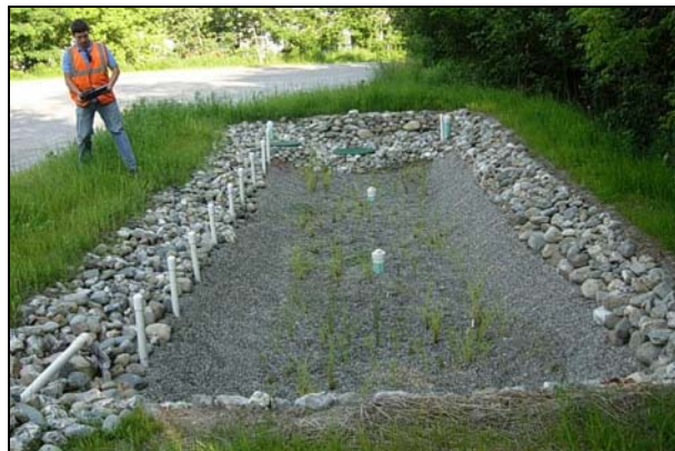
An example of a capital project construction (a gravel wetland) that was paid for by the stormwater utility in South Burlington, Vermont.
