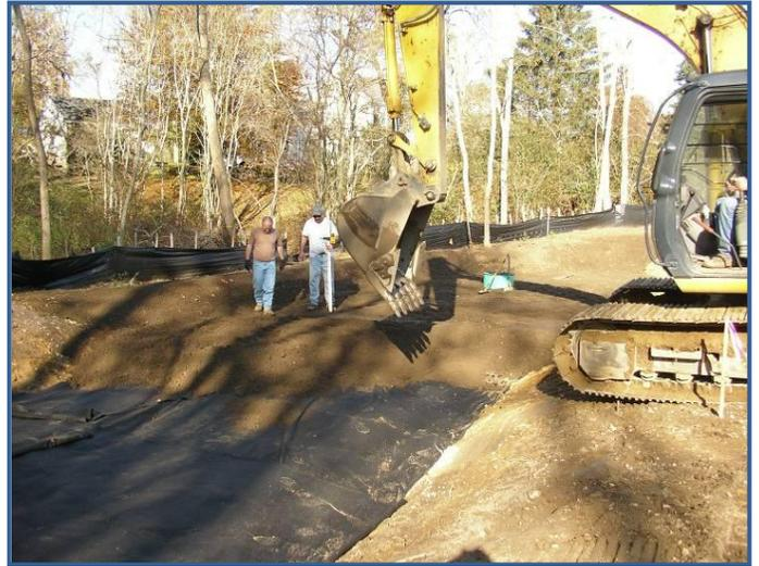
**Figure 4.** As an example of a priority retrofit taken to final design and construction, this shows the installation of a bioretention facility at a nature center in Massachusetts.
