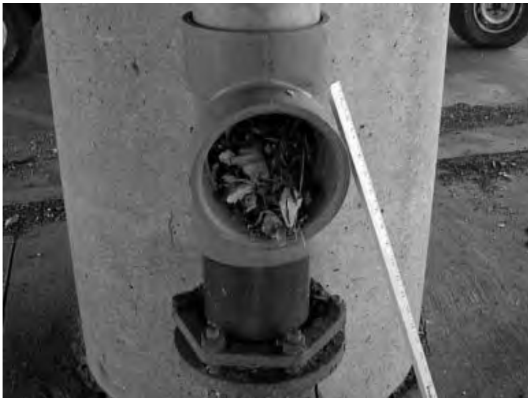
Figure 1. Example of poorly maintained stormpipe from Interstate I-190 overpass. Note pipe is completely clogged with sediment and debris.
