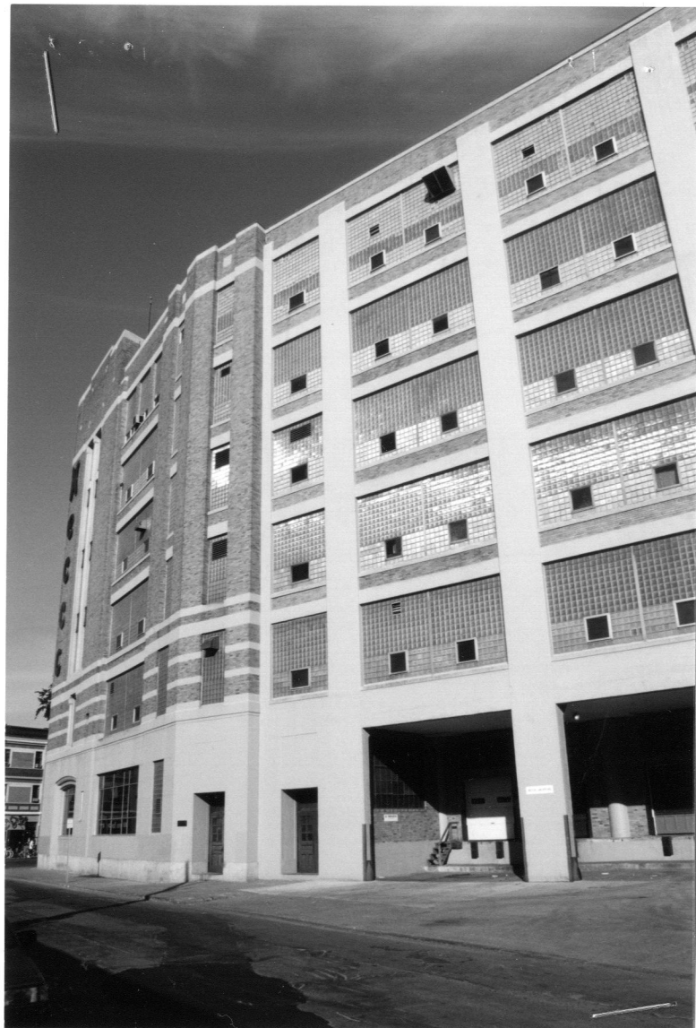
LANDSDOWNE ST (W) FACADE LOOKING NORTH
