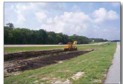
Figure 37. Recycling sediment along a highway
