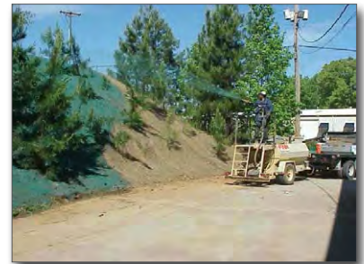
Figure 5. Hydroseeding the slope
