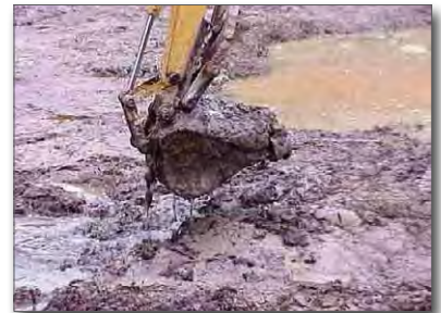
Figure 36. Removing stiffened sediment from a sediment basin
