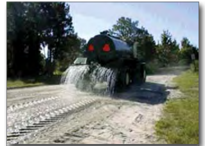
Figure 11. Water truck applying dissolved polymer flocculant
