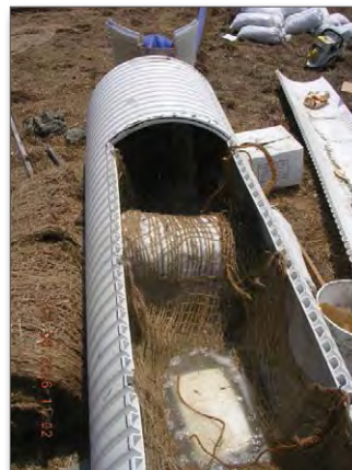
Figure 20. Split pipe with polymer blocks
