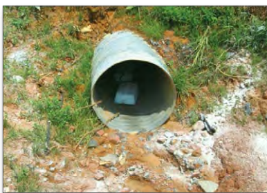
Figure 39. Polymer block in a construction site culvert
