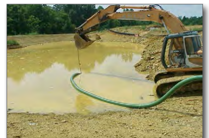
Figure 14. Sediment basin to be dewatered
