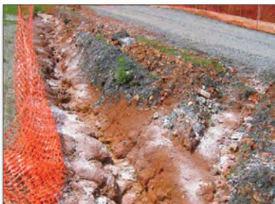
Figure 38. Eroding gully on a construction site
