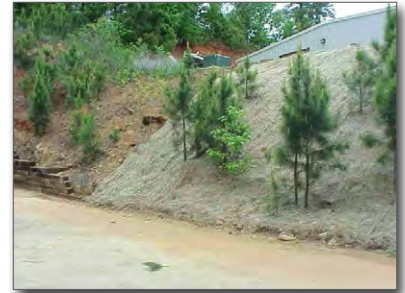
Figure 4. Slope covered with floc collection matting
