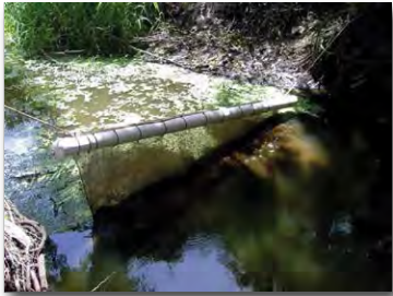
Figure 29. Particle curtain in a canal
