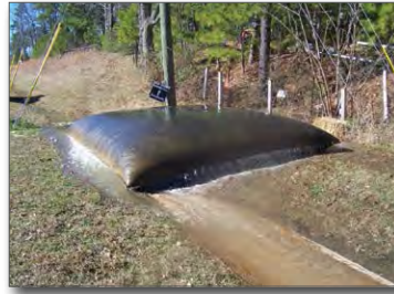
Figure 34. Sediment bag and its treatment ditch
