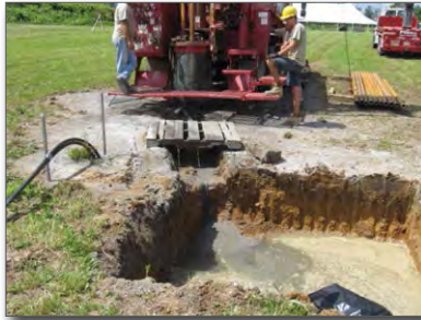
Figure 7. Drilling rig and settling pit
