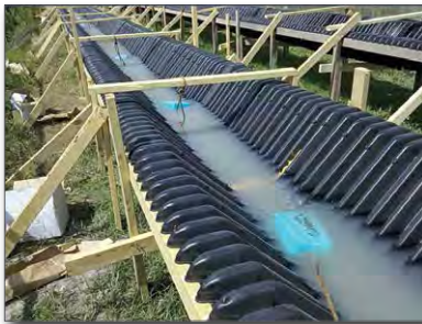
Figure 17. HDPE treatment ditch liner
