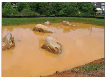
Figure 40. Sediment pond before BMPs were installed
