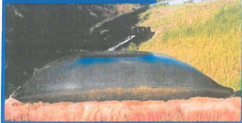
Hillside Installation on Straw Underlayment
