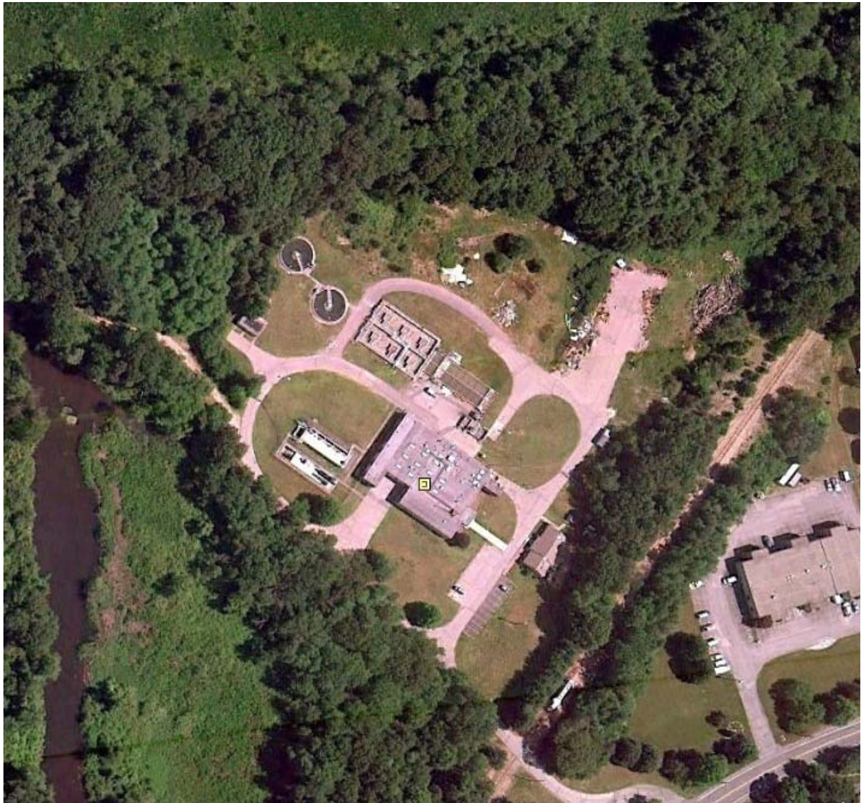
Figure 2. Aerial Photo of Medfield Wastewater Treatment Facility
