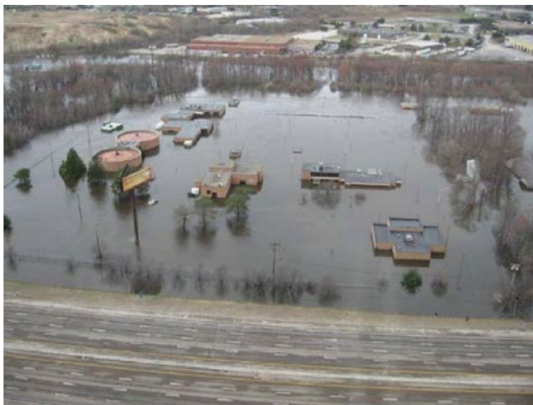
Figure 1: The flooded Warwick wastewater facility on Wednesday, March 31, 2010. (State of Rhode Island)
